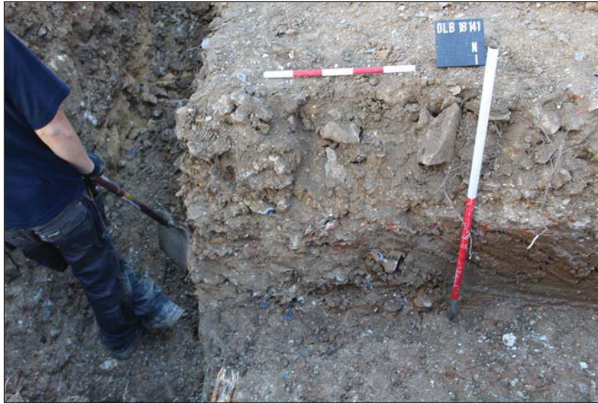
Plate 3. East side of demolition backfill (3) cutting tile at top of sunken construction (cut 2), looking north east, Scales 0.5m and 1m.
