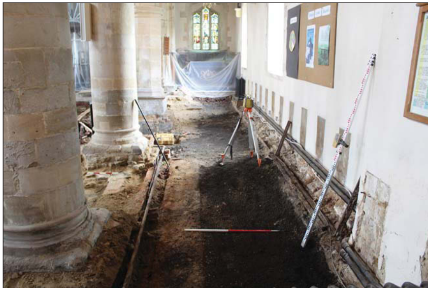
Plate 2. Formation level reached in south aisle, looking east, Scales: 1m.
