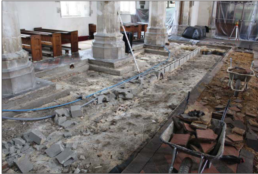
Plate 1. Extent of 1980's floor works and north arcade.
