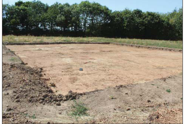
Plate 2. Area B, looking west north west, Scales: 2x1m.
