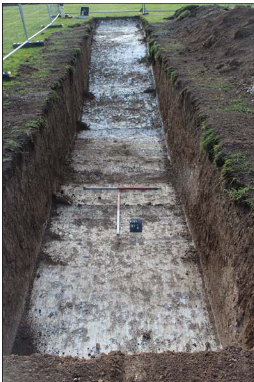
Plate 7. Trench 7, looking south, Scales: 1m
