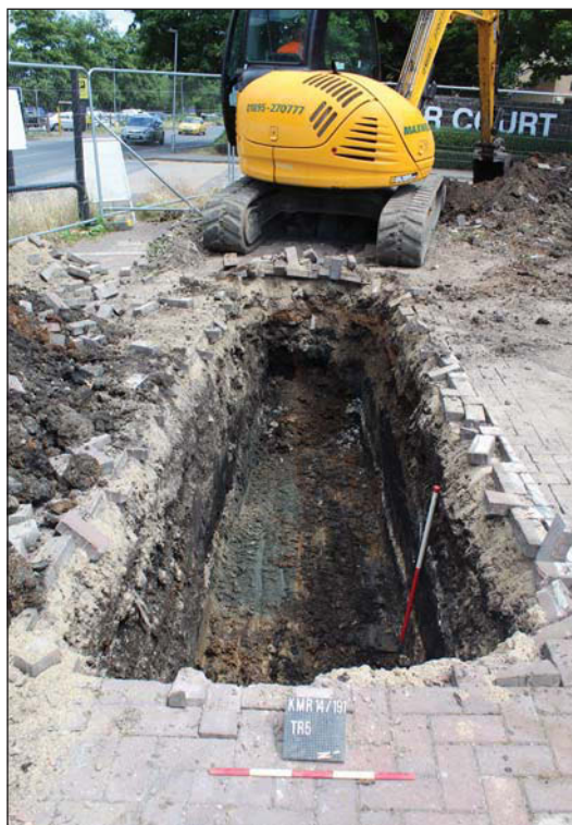
Plate 2. Trench 5, looking east, Scales: horizontal 0.5m, vertical 1m.
