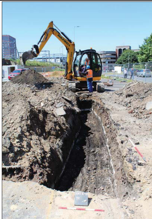
Plate 1. Trench 1, looking east, Scales: 1m and 0.5m.
