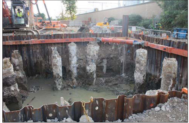
Plate 2. The western core excavation, showing alluvial deposits and groundwater, looking south-east.
