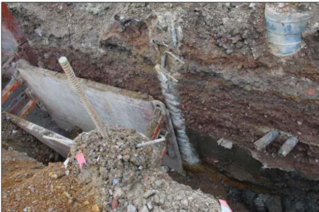
Plate 3. Excavations at the western end of the site showing layers of made ground overlying the alluvial clay, looking west.
