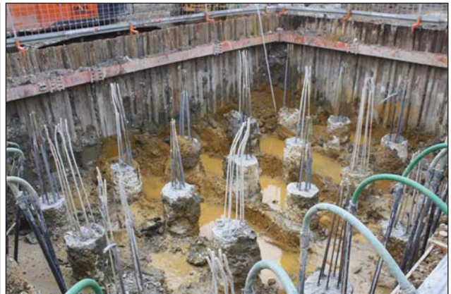
Plate 4. The eastern core excavation, showing gravel deposits, looking south-west.
