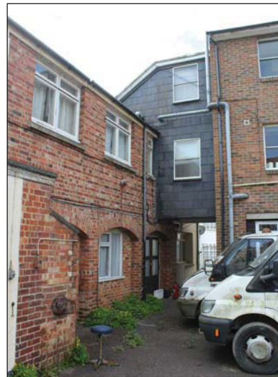
Plate 4. General view of west side of building, looking South-south-east.
