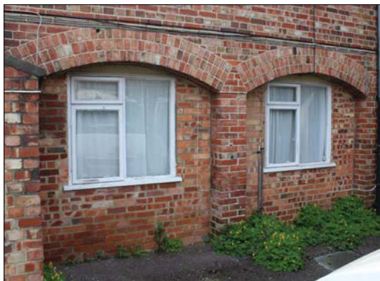
Plate 3. Close-up of west side of building, looking East.
