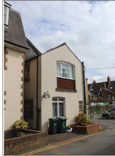
Plate 6. General view of west and south sides of building, looking North-east.
