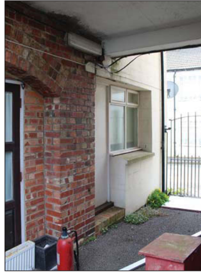
Plate 2. Close-up of west side of building, looking South-east.
