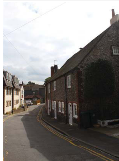
Plate 8. General view down North Road, looking East.
