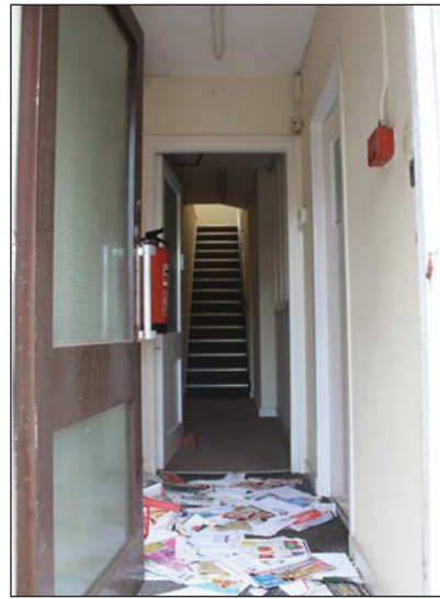
Plate 10. View through front door towards corridor G1, looking South.
