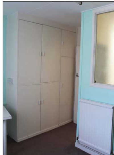
Plate 16. General view of room F5, looking North-west.
