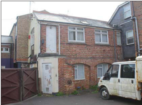
Plate 7. General view of north and west sides of building, looking South-east.
