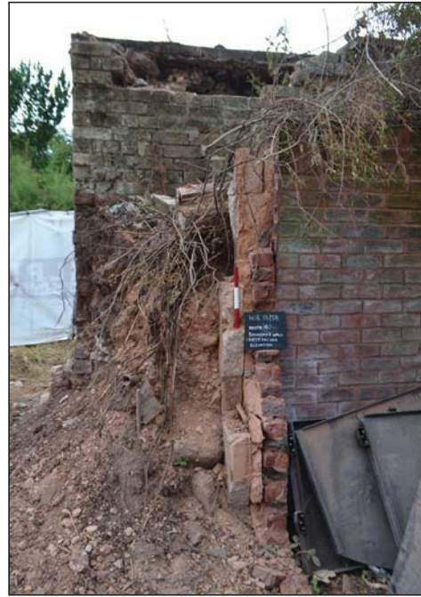
Plate 10. Boundary wall, during demolition, looking west, Scale: 0.3m.
