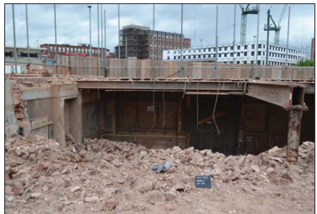
Plate 2. Honiton Inn during demolition, looking north-northwest.
