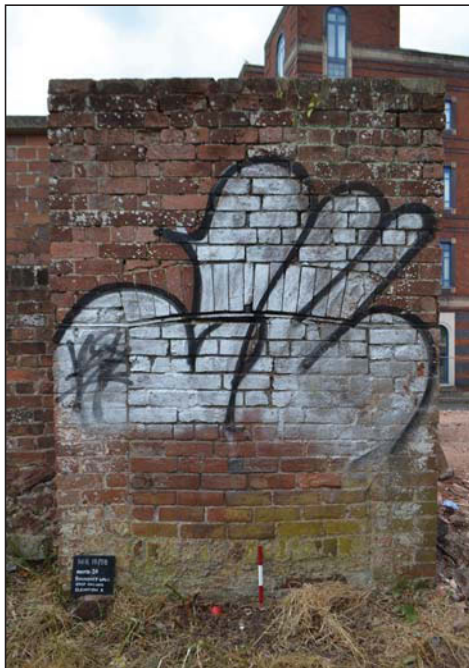
Plate 3. Boundary wall (north end), looking west, Scale: 0.3m.
