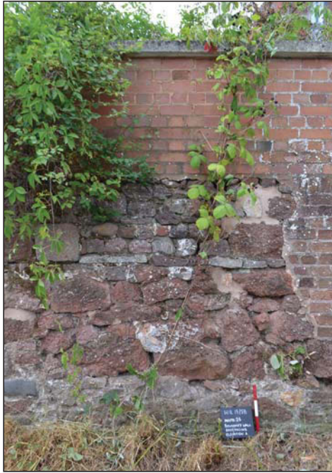
Plate 5. Boundary wall, looking west, Scale: 0.3m.
