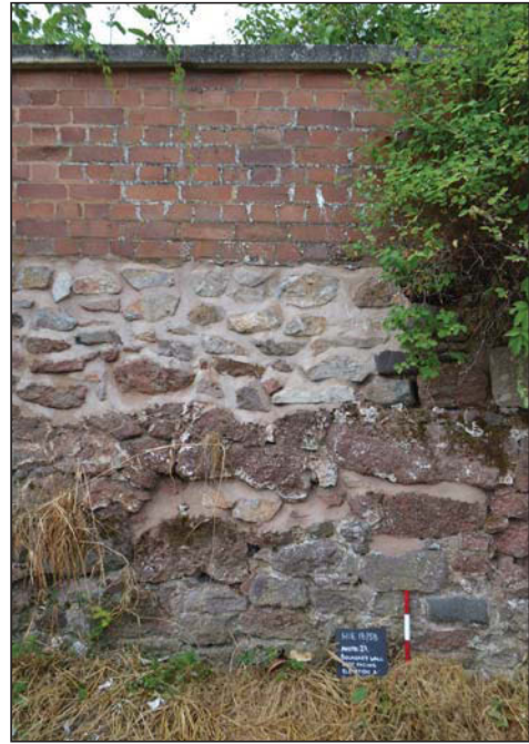
Plate 6. Boundary wall, looking west, Scale: 0.3m.
