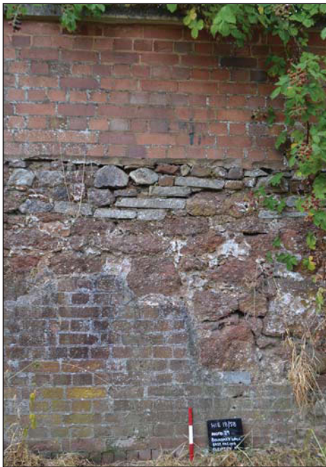
Plate 7. Boundary wall, looking west, Scale: 0.3m.
