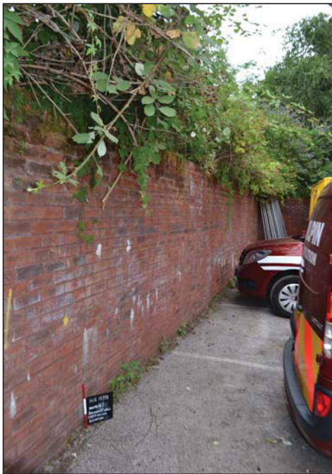
Plate 11. West face of Boundary wall, looking south, Scale: 0.3m.
