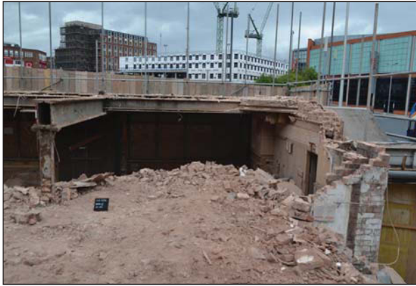
Plate 1. Honiton Inn during demolition, looking north-northeast.
