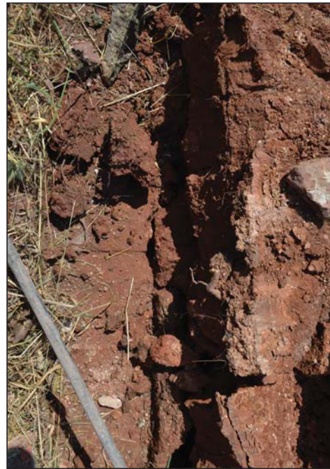
Plate 14. Boundary wall after demolition, foundation remains, looking west, Scale: 0.3m.
