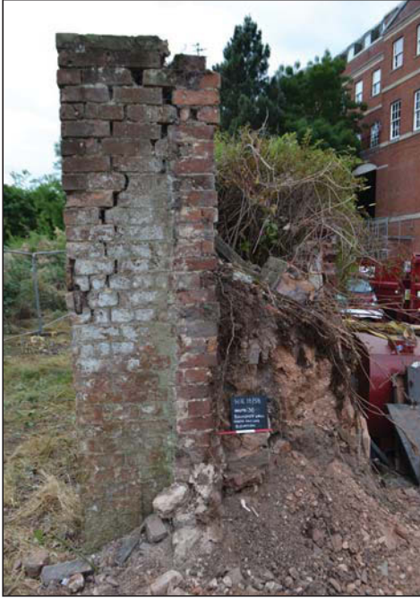
Plate 9. Boundary wall (west end) during demolition, looking west, Scale: 0.3m.
