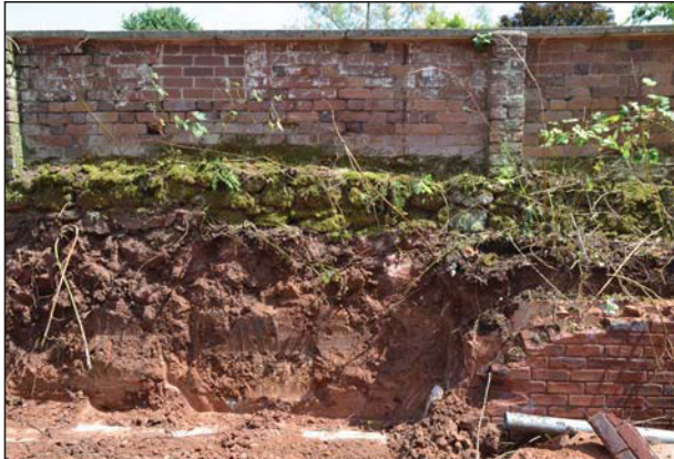
Plate 13. Boundary wall (west end) during demolition, looking east, Scale: 0.3m.
