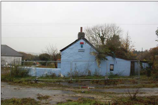
Plate 3. Exterior, NE facing side elevation, looking SW, Scales: 2 x 1m
