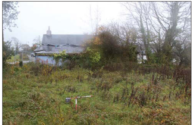
Plate 4. Exterior, rear elevation, looking SE, Scales: 2 x 1m.
