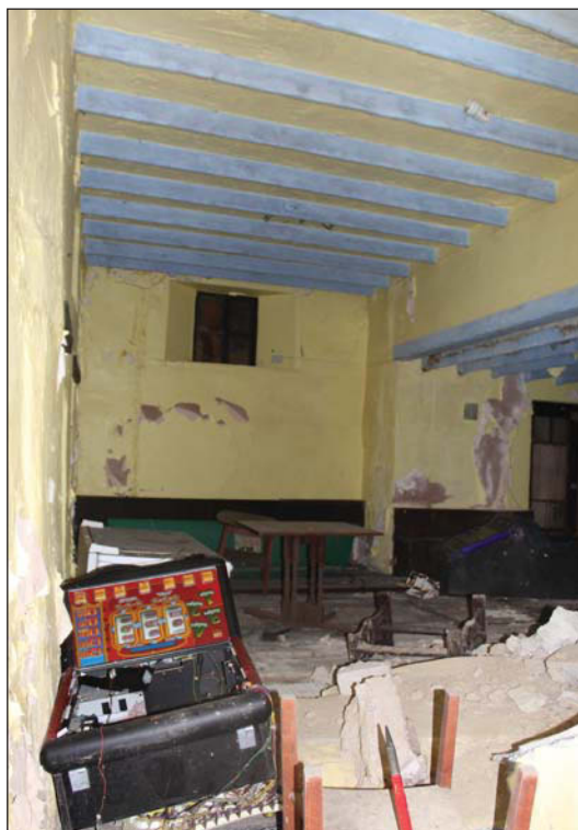
Plate 10. Interior, Room 1 and 2, looking NNW.
