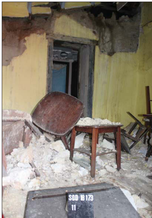
Plate 8. Interior, Room 1, looking NNW. Scales: 2 x 1m.
