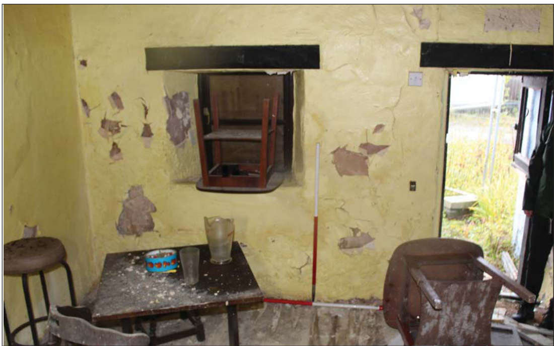
Plate 12. Interior, Room 1, Looking SE. Scales: 2 x 1m
