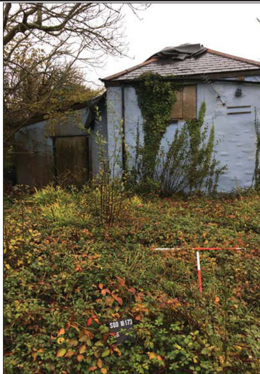
Plate 5. SW facing side elevation, looking NE, Scales: 2 x 1m.
