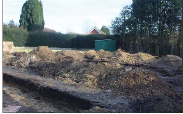
Plate 2. General view of site, looking North-east.
