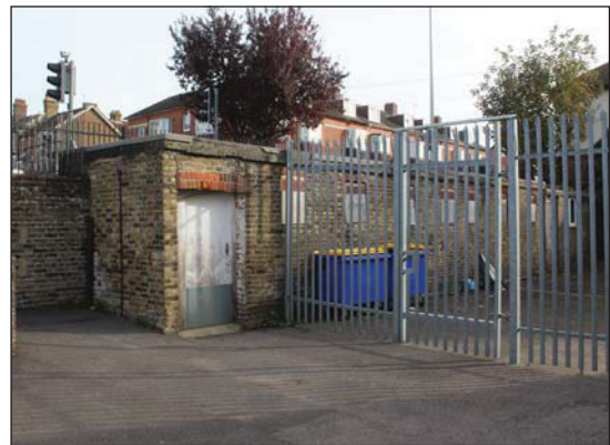
Plate 8. General view of Building C, looking North-east.
