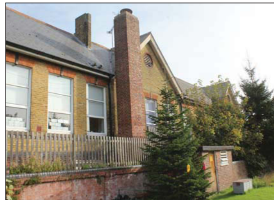
Plate 16. General view of Building A from garden area, looking North-east.
