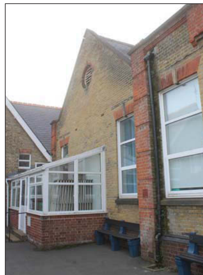
Plate 4. Vestibule A19, linking Buildings A and B, looking South South-east.
