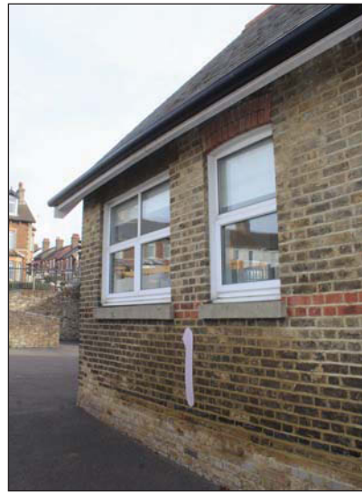
Plate 6. General view of Building B, looking North-east.
