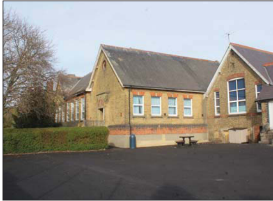
Plate 13. General view of Buildings A and B, looking North-west.
