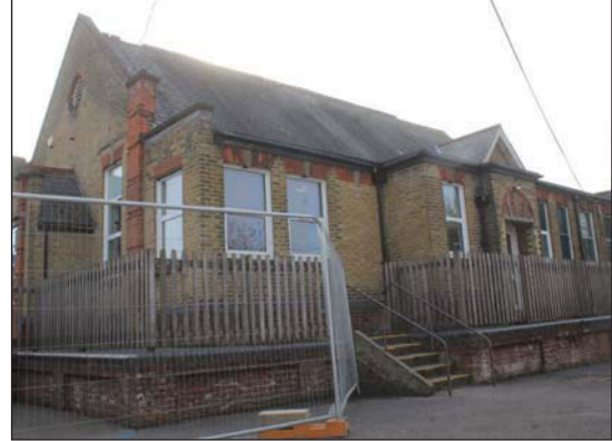
Plate 18. General view of Building A, looking South South-east.
