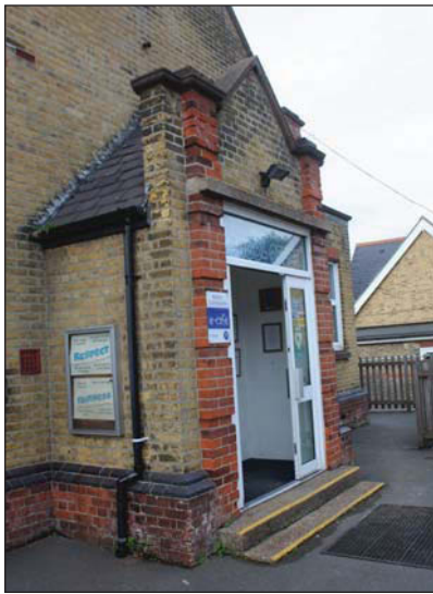
Plate 1. General view of main entrance to Building A, looking West.
