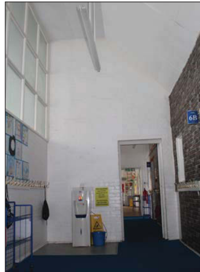
Plate 40. General view of Lobby / Corridor B1, looking North North-east.
