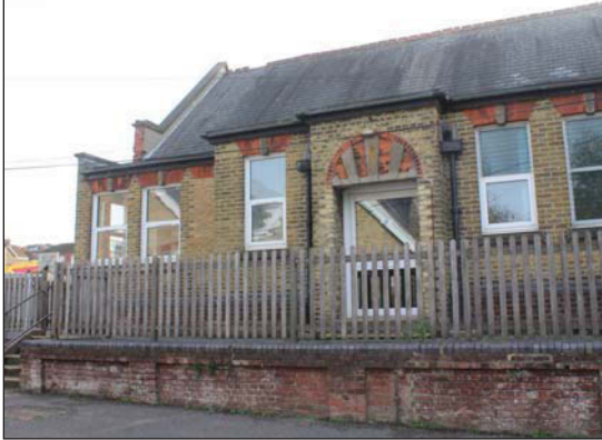
Plate 17. General view of Building A, looking East South-east.
