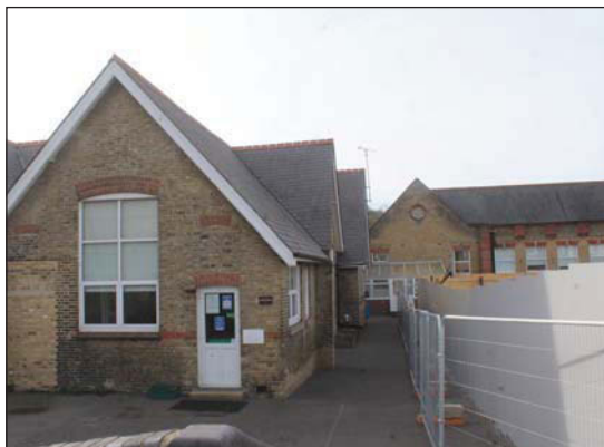
Plate 7. General view of Buildings A and B, looking South South-west.
