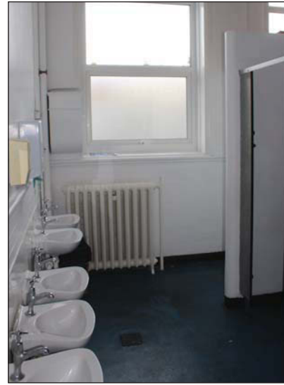
Plate 30. General view of Girl's WC, looking North North-east.
