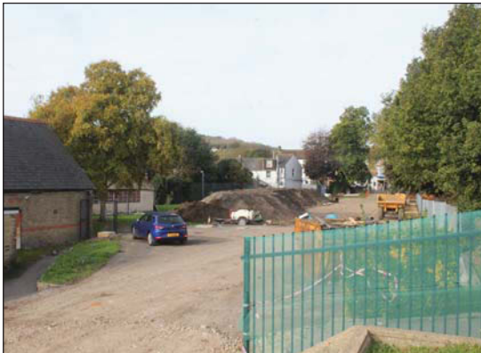
Plate 23. General view of playing field (Building D to left), looking West.
