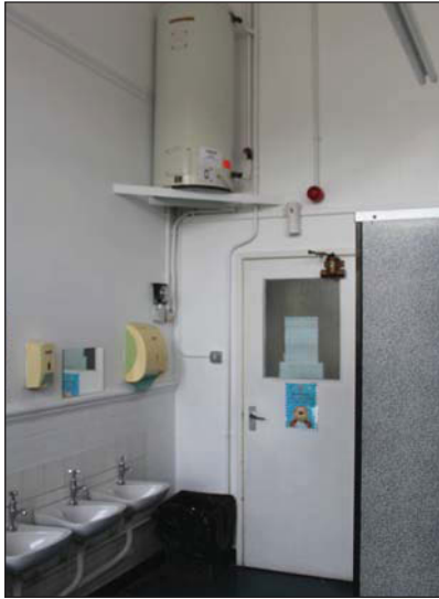
Plate 33. General view of Boy's WC A15, looking South South-west.
