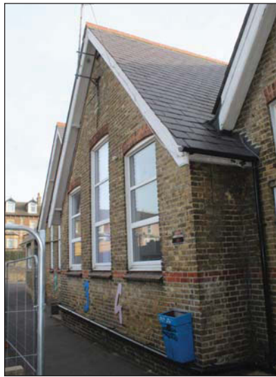
Plate 5. General view of Building B, looking North-east.
