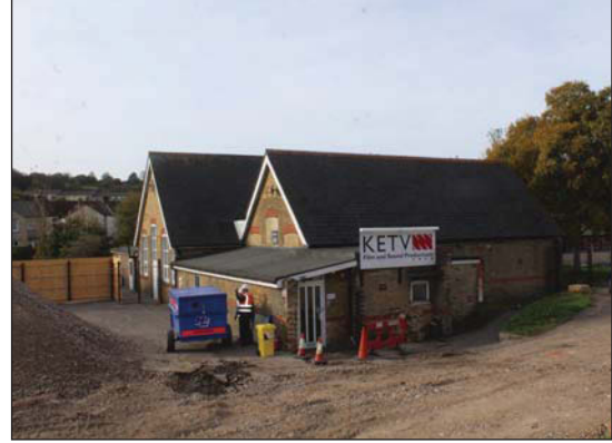
Plate 22. General view of Building D, looking South-west.
