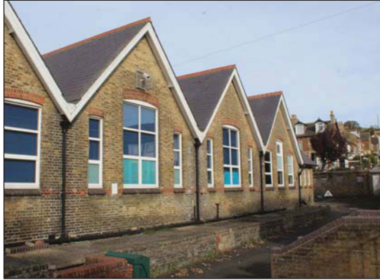
Plate 9. General view of Building B (Building C in background), looking North.
