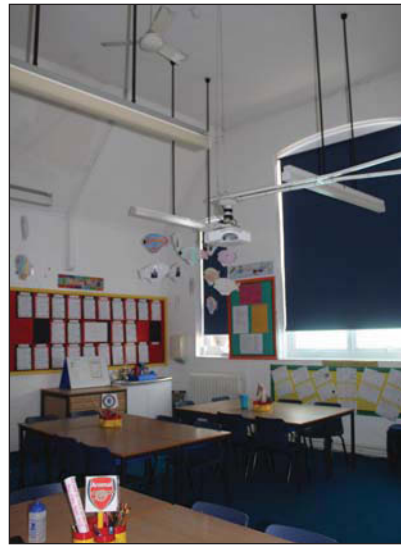
Plate 38. General view of Classroom B2, looking South South-east.
