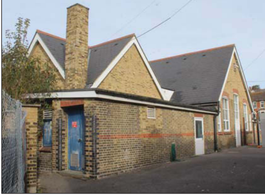
Plate 21. General view of Building D, looking North.
