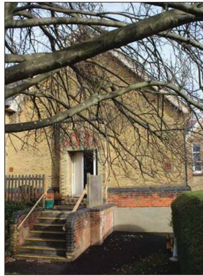
Plate 14. General view of Building A from garden area, looking North.
