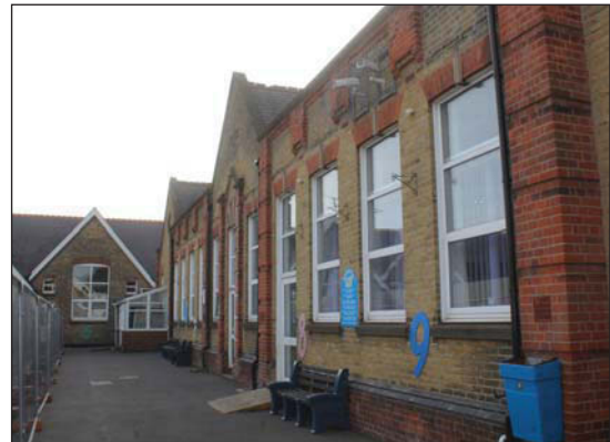
Plate 2. General view of Building A (Building B in background), looking South-east.
