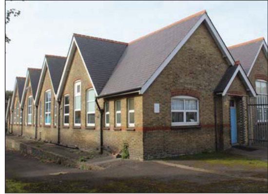
Plate 10. General view of Building B, looking South-west.
