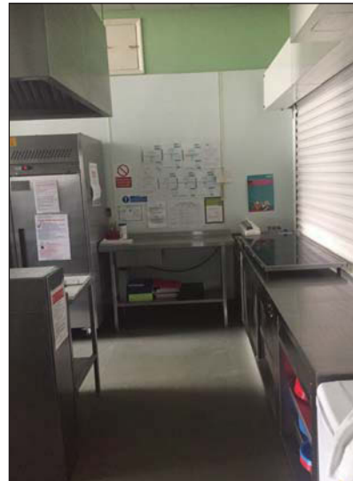
Plate 48. General view of Kitchen B13, looking South South-west.
