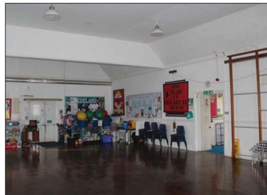
Plate 36. General view of Assembly Hall / Gym A18, looking South-west.
