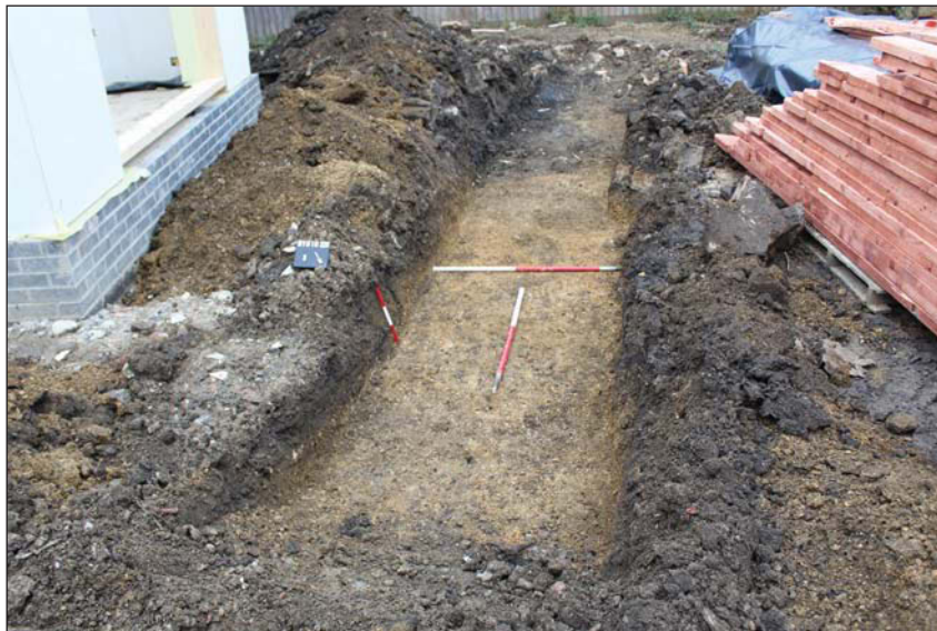
Plate 2. Trench 3, looking south east, Scales: horizontal 1m x2, vertical 0.3m.
