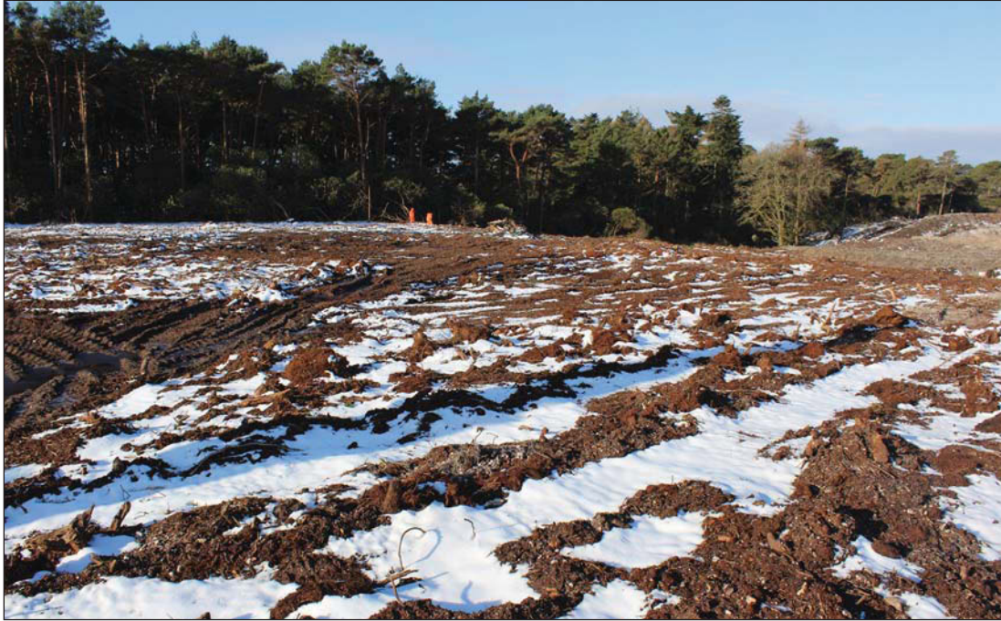
Plate 3. Site looking west after tree felling and stump removal
