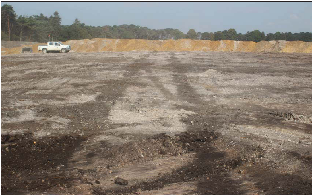
Plate 6. Ruts 2 and 3 looking west
