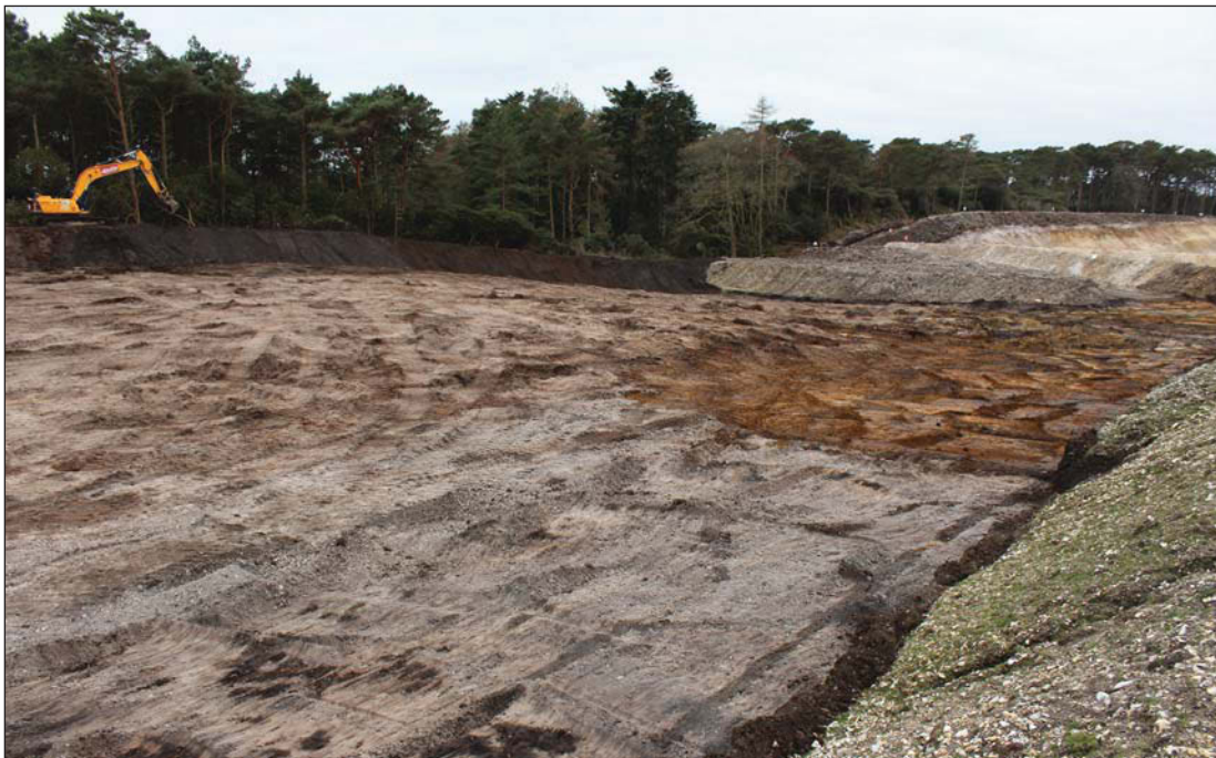
Plate 4. Site looking west whilst topsoil stripping
