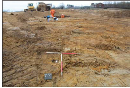
Plate 2: General view of site after stripping
