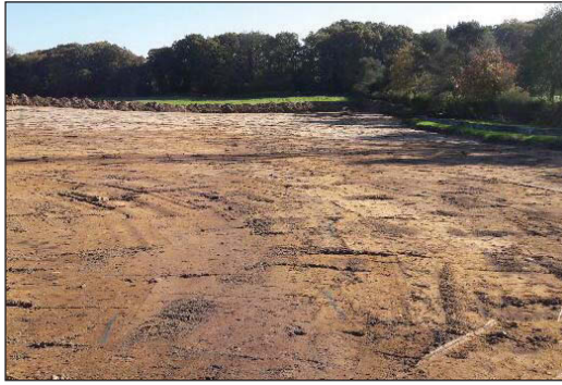
Plate 1: General view of site after stripping
