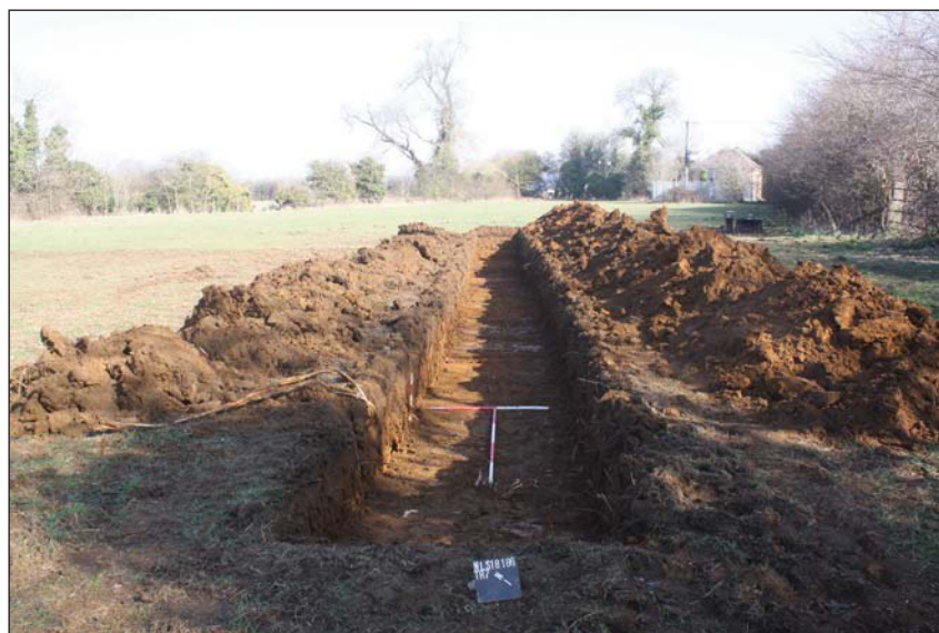
Plate 4. Trench 7, looking north east, Scales: horizontal 2m and 1m, vertical 0.5m.
