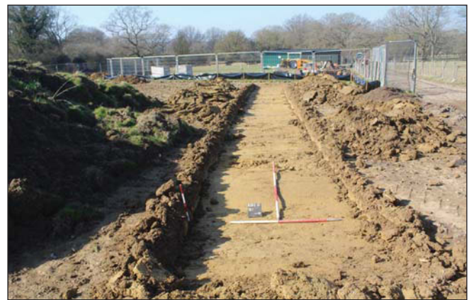
Plate 4. Trench 7, looking West-north-west. Scales: 2m, 1m and 0.50m.
