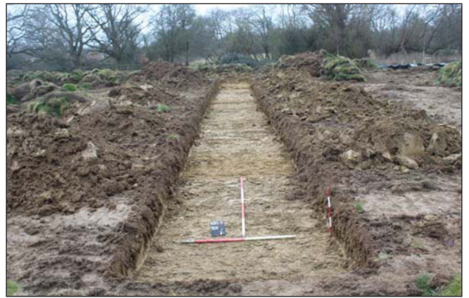
Plate 16. Trench 36, looking South. Scales: 2m, 1m and 0.50m.
