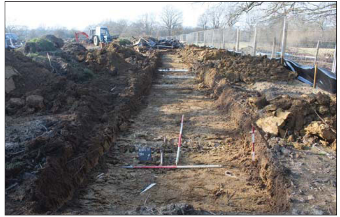
Plate 2. Trench 4, looking West-north-west. Scales: 2m, 1m and 0.50m.
