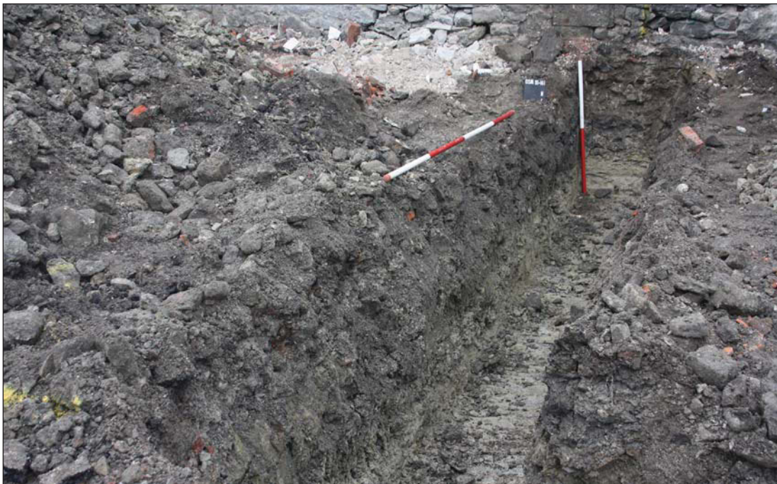
Plate 2. Existing and excavated footings, looking SE, Scales: 1m and 2m.
