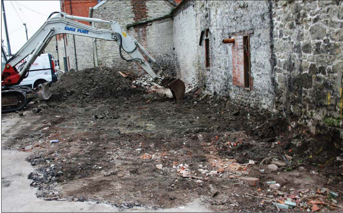
Plate 1. Area footings, looking SE
