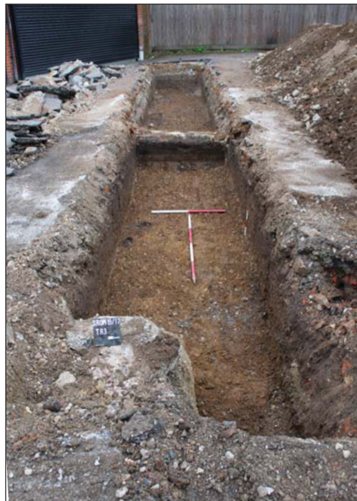
Plate 2. Trench 3, looking east, Scales: horizontal 2m and 1m, vertical 0.3m.
