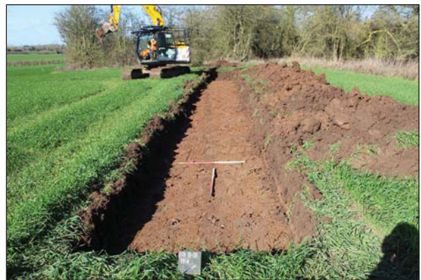
Plate 6. Trench 4, looking NW, Scales: 2x1m.
