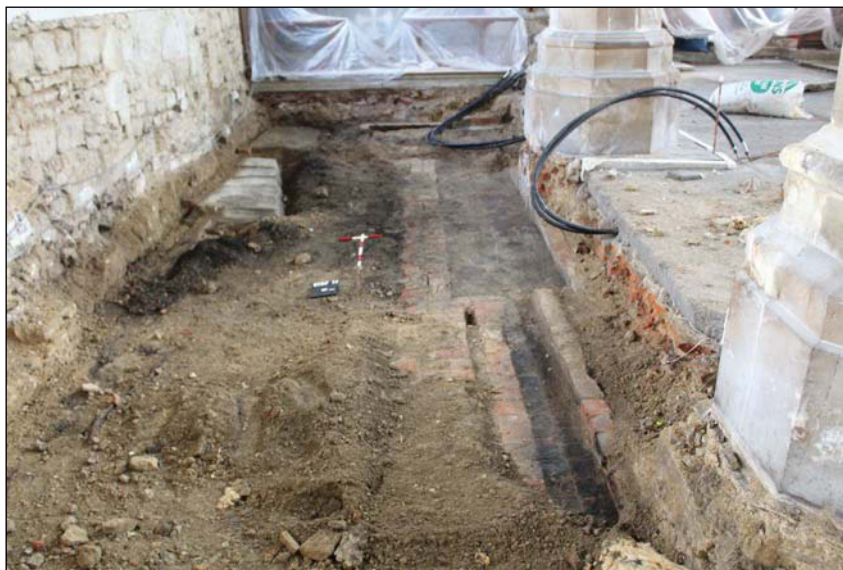
Plate 4. Bases of Victorian duct and pipe system and grave slabs, looking east, Scales: 0.5m and 0.3m.
