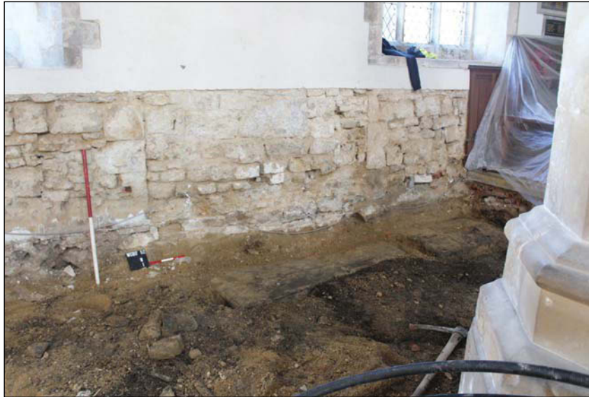
Plate 3. Exposed stone construction of north aisle wall, looking north, Scales: 1m and 0.3m.
