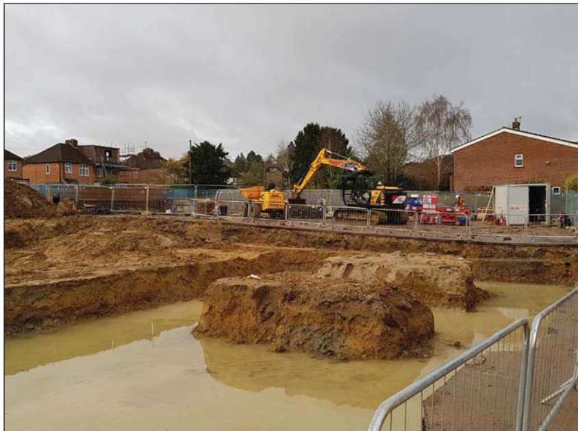
Plate 4. Area F, excavated footings, looking south west.
