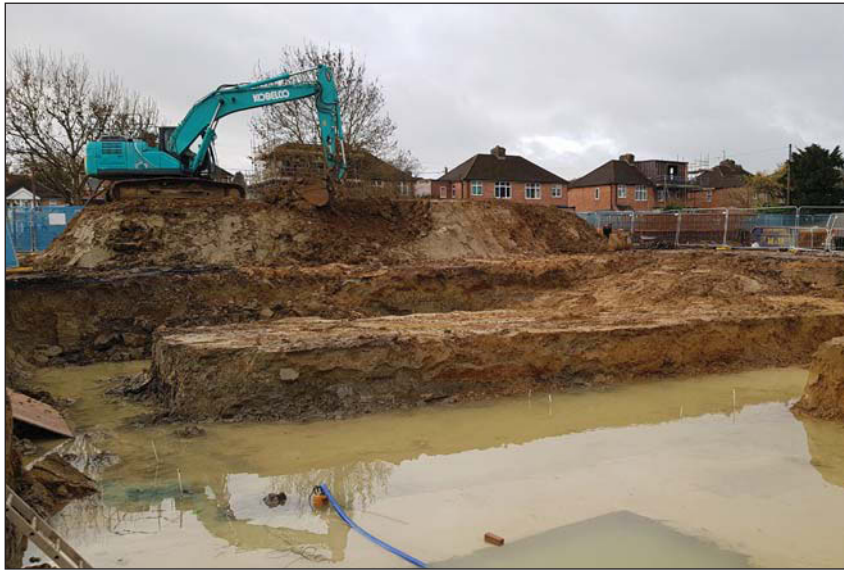
Plate 3. Area F, Excavated footings, looking south south west.
