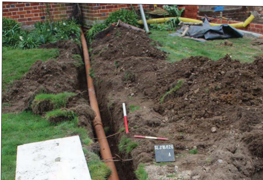
Plate 4. Service trench, looking N, Scales: 1m and 0.30m.
