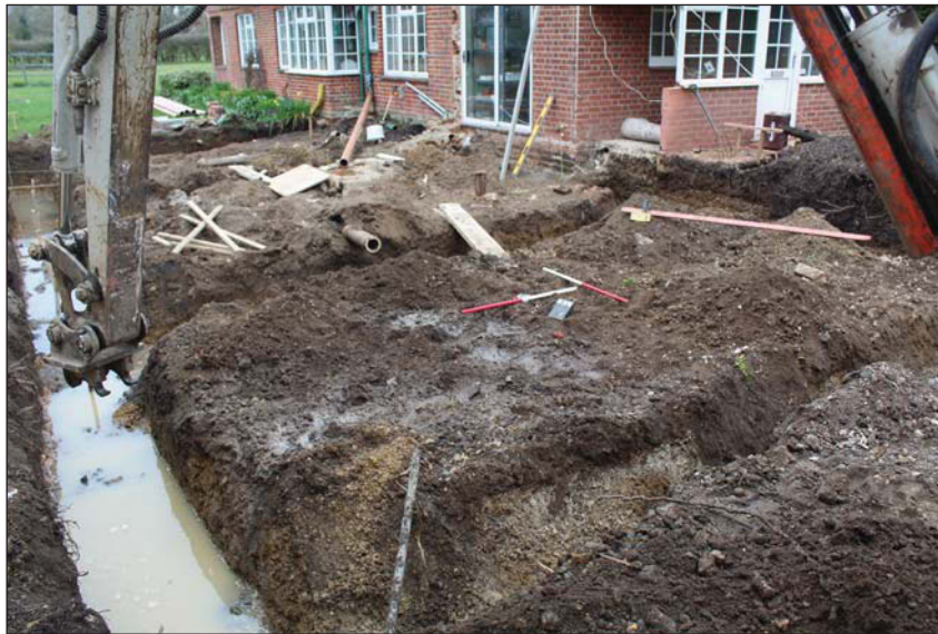
Plate 3. General view of the footing trenches, looking W, Scales: 2x1m.
