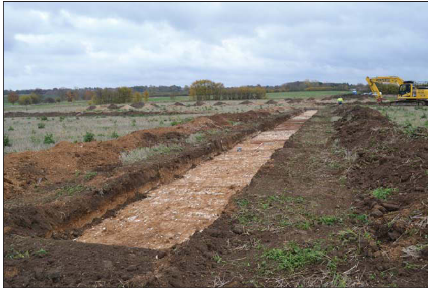
Plate 1. Trench 20, looking north east, Scales: horizontal 2m and 1m, vertical 0.5m.
