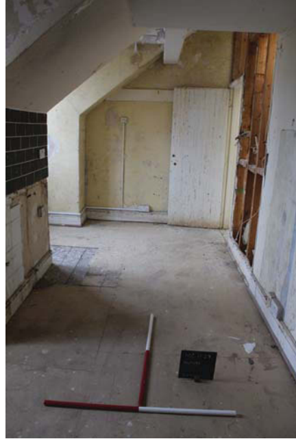
Plate 52. Room 7, looking south.
