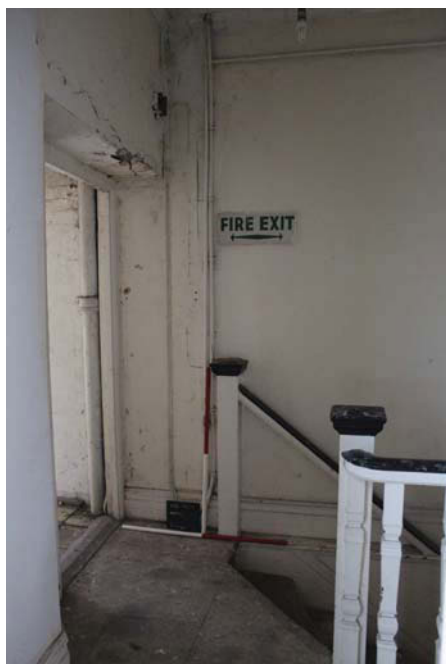
Plate 29. Detail of top of stairs (first floor corridor), looking south-east.
