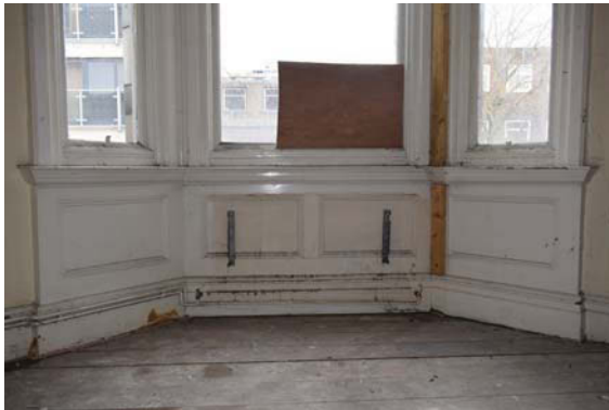
Plate 37. Detail of window panel, room 3, looking west.
