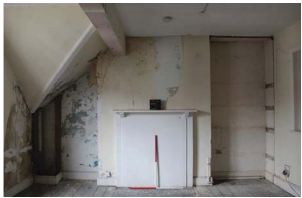
Plate 50. Room 8 fireplace detail, looking north.
