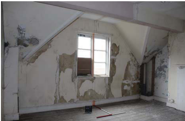
Plate 49. Room 8, view north-west to window.
