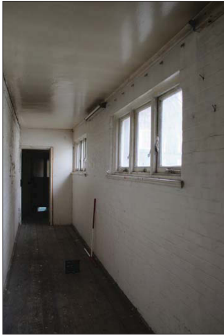
Plate 23. Link walkway, oblique view of south wall, looking south-east.
