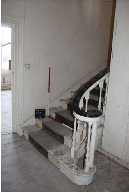
Plate 31. First floor corridor, stair detail, looking north-west.
