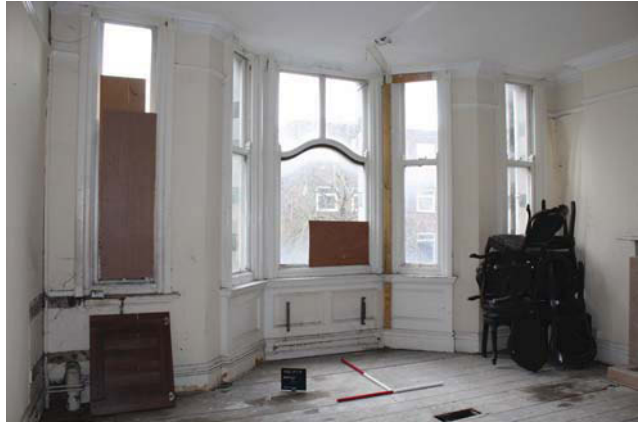
Plate 36. Windows, room 3, looking north-west.
