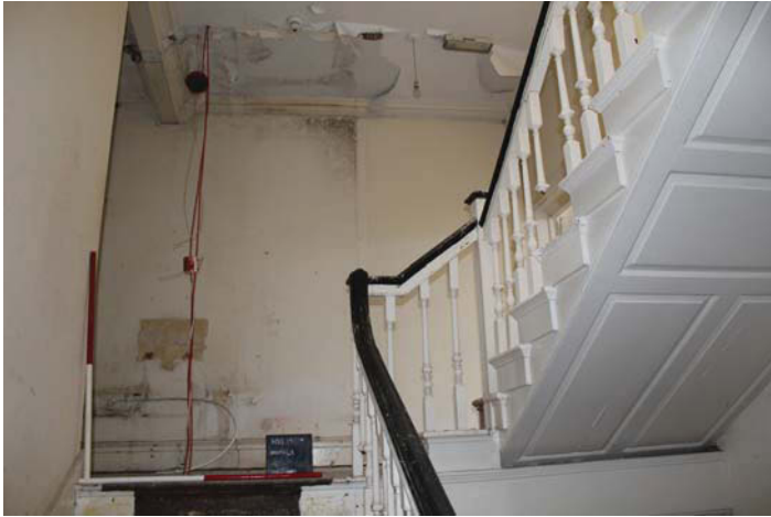
Plate 39. Stairs, second floor landing, looking north.
