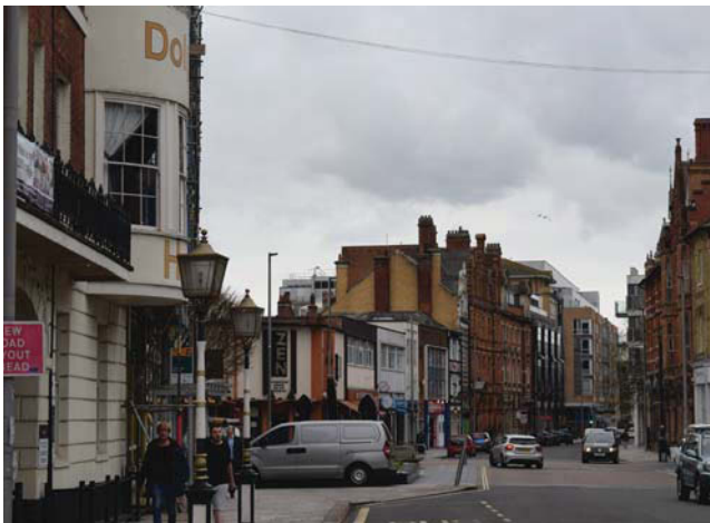
Plate 15. North gable wall, facing S.
