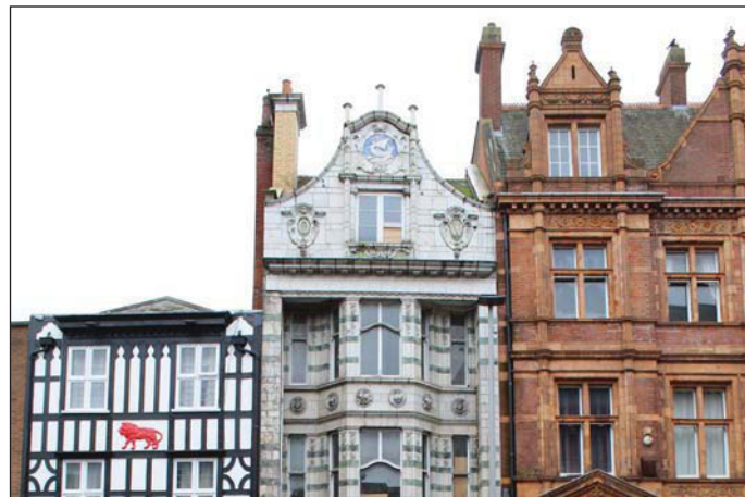
Plate 4. 1st floor window detail, looking east
