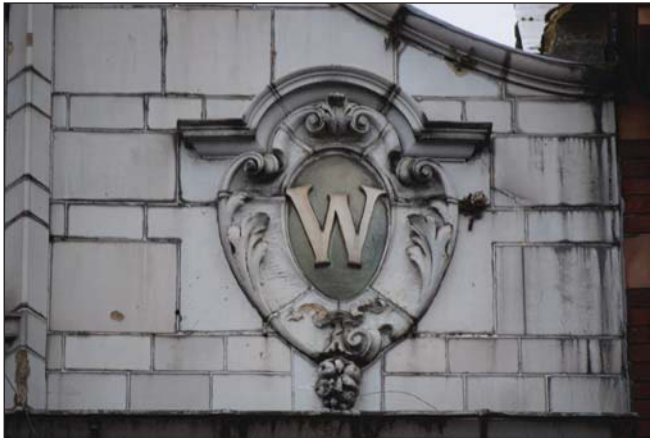
Plate 13. 'W' detail, looking east
