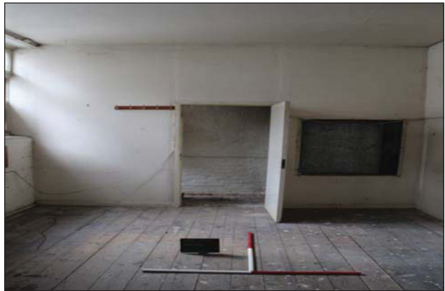
Plate 24. Stud wall dividing room 1, looking south.
