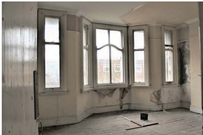
Plate 41. View north-west to windows, room 4..
