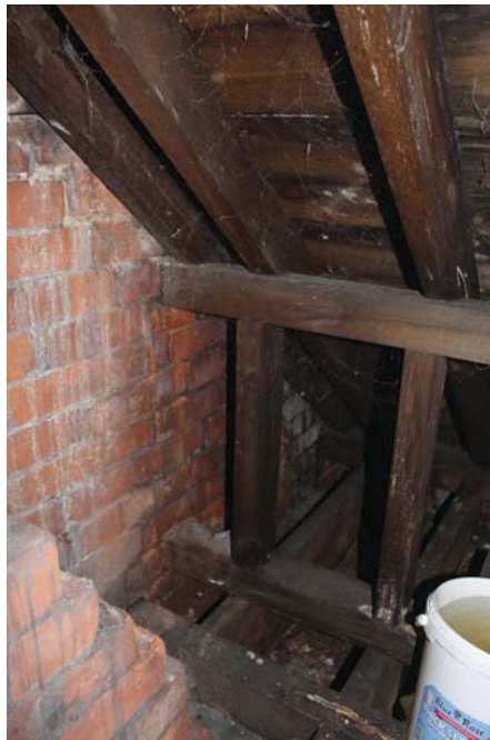
Plate 53. Room 7 north gable wall and chimney breast, looking north-east.
