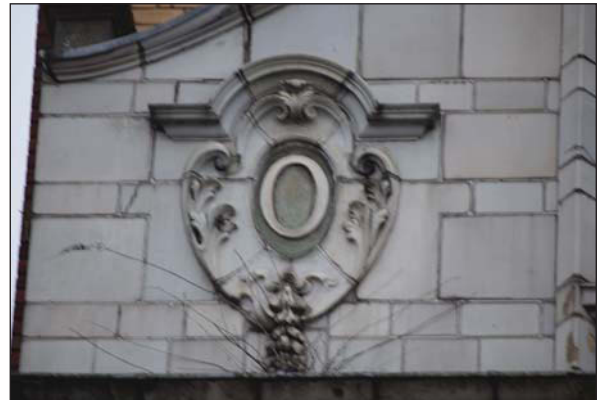
Plate 12. 'O' detail, looking east
