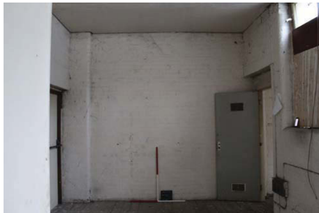
Plate 26. South wall of room 1, looking south.
