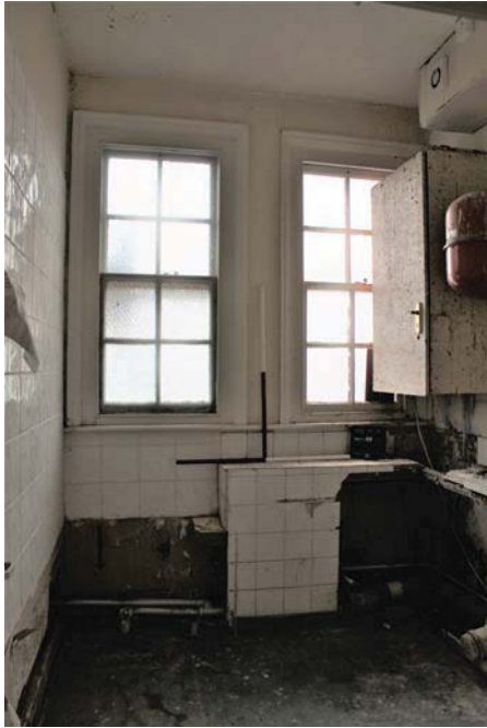
Plate 43. Room 5, looking east to windows.
