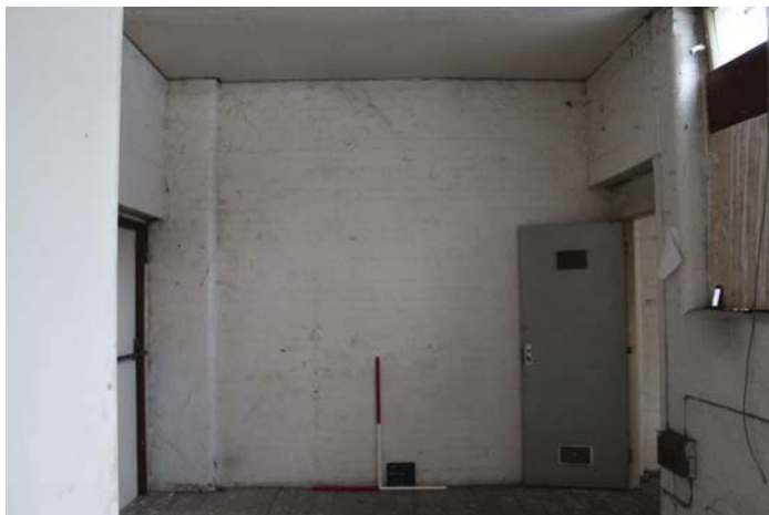
Plate 27. Stairwell, view to north wall.
