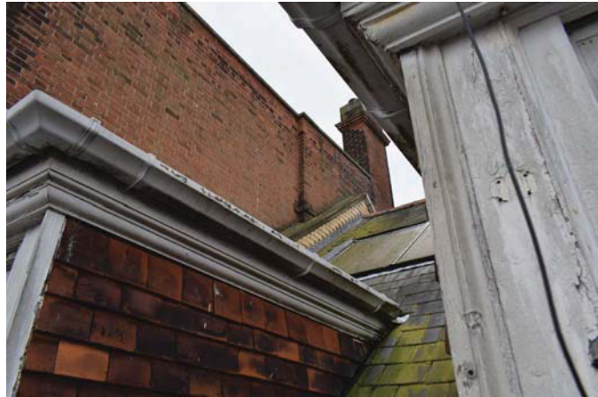
Plate 18. South gable detail. SW facing
