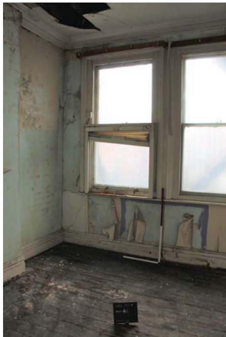
Plate 45. Room 6 looking north-east to windows.
