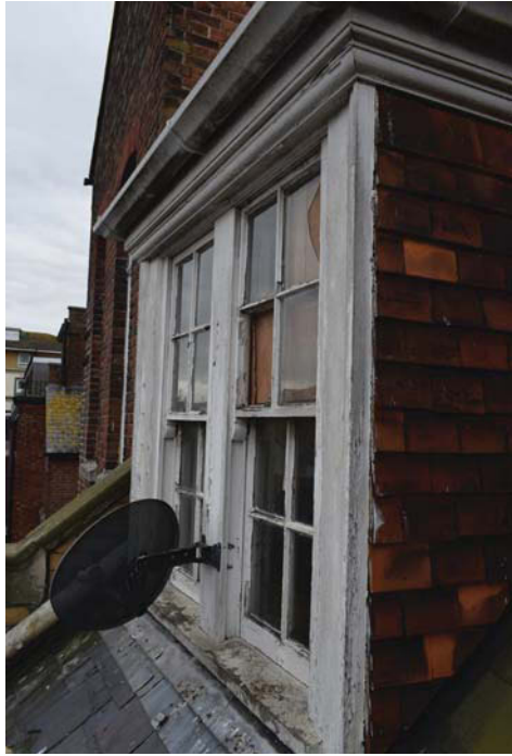
Plate 17. Dormer window detail. SW facing
