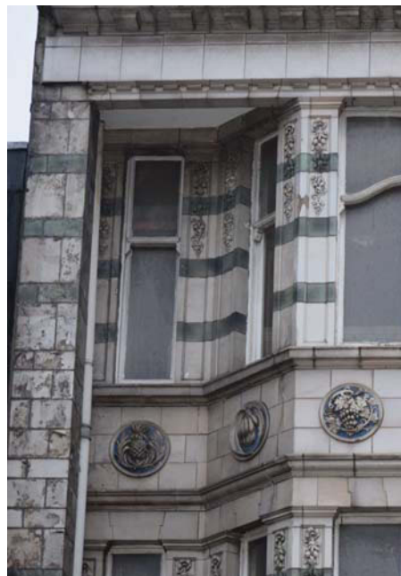
Plate 22. 1st floor. Link walkway opening. E facing.
