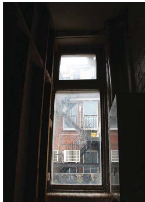
Plate 16. View through window to rear of 56 High Street. W facing.
