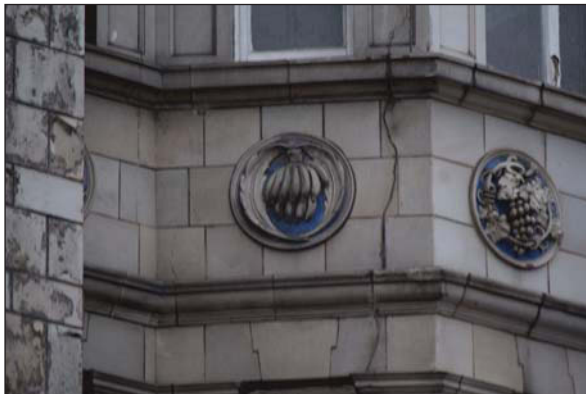
Plate 7. North roundel detail on bay window, looking south east
