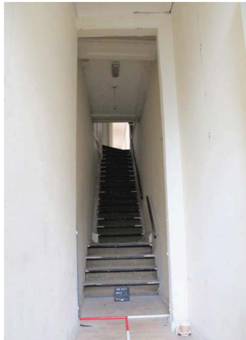
Plate 20. Ground floor corridor. Stair detail. E facing.
