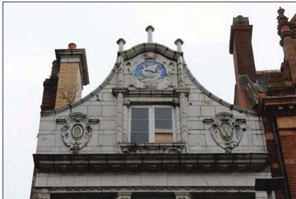
Plate 11. Third floor detail of High Street elevation, looking east
