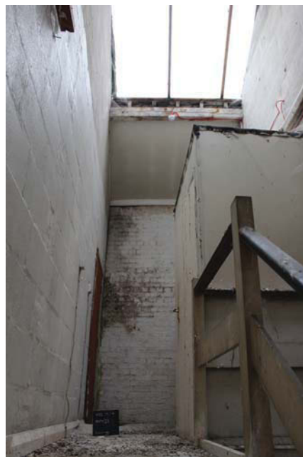
Plate 28. Stairwell, view to south wall and skylights.
