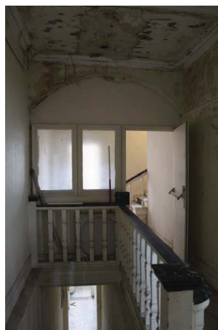
Plate 30. First floor corridor, stair baluster detail and arch, looking west.
