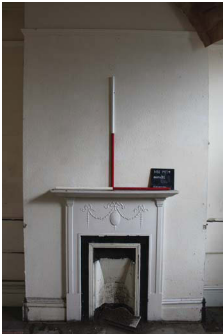
Plate 33. Room 2, fireplace detail, looking north.
