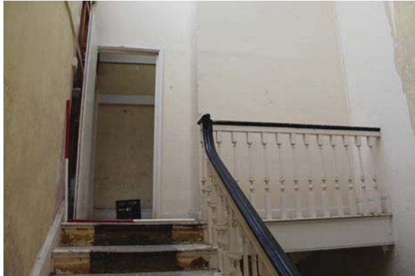
Plate 47. Third floor stair detail, looking north.
