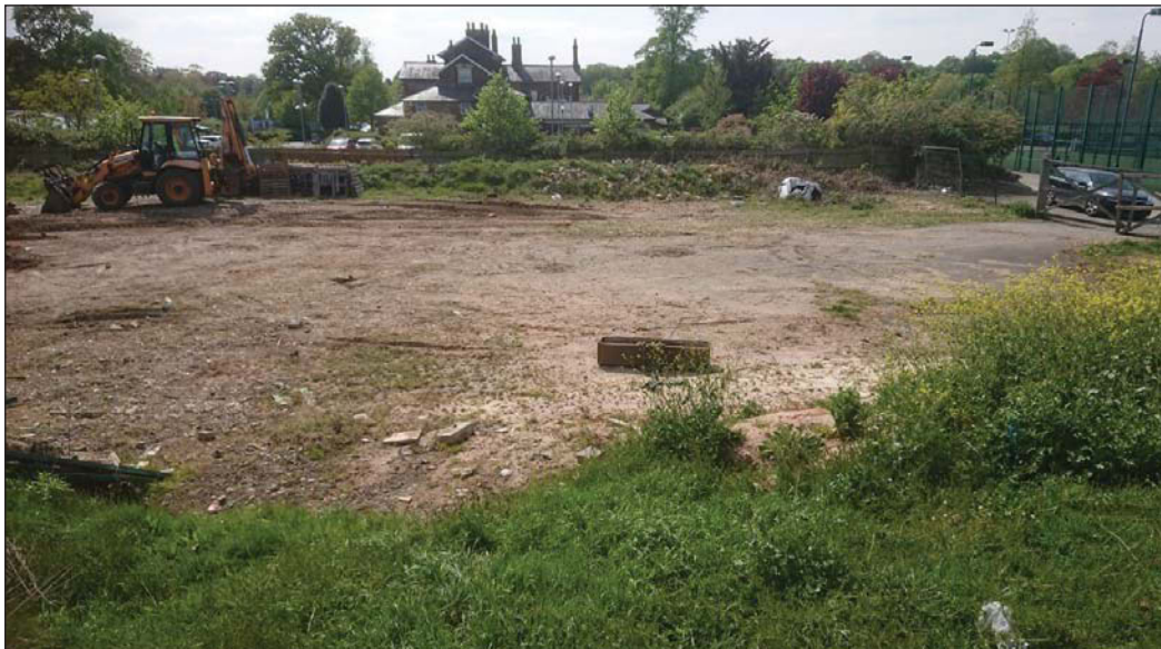
Plate 8. General view of site looking west towards Stafferton Lodge.
