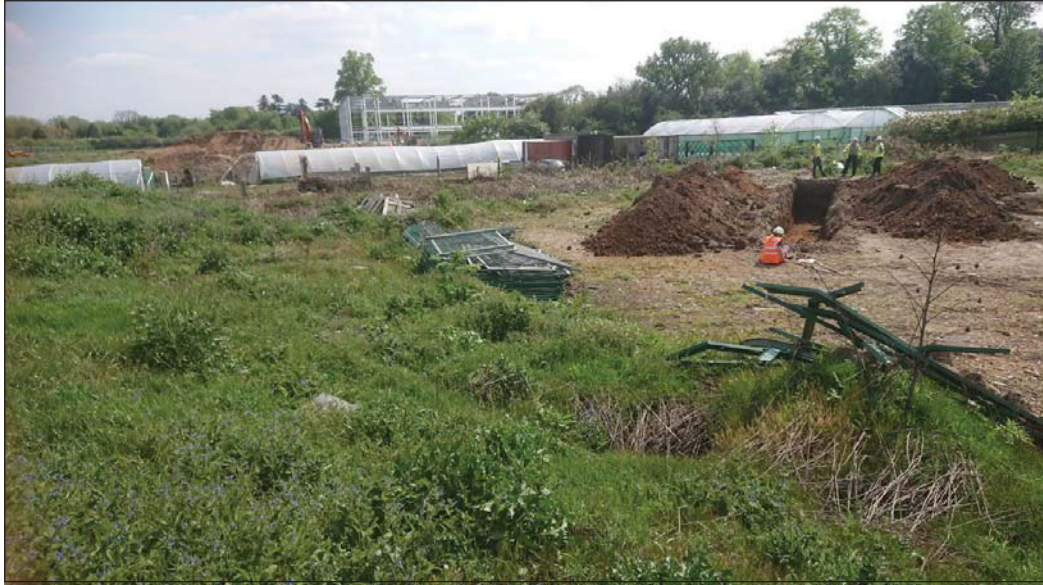
Plate 7. General view of site, looking south.
