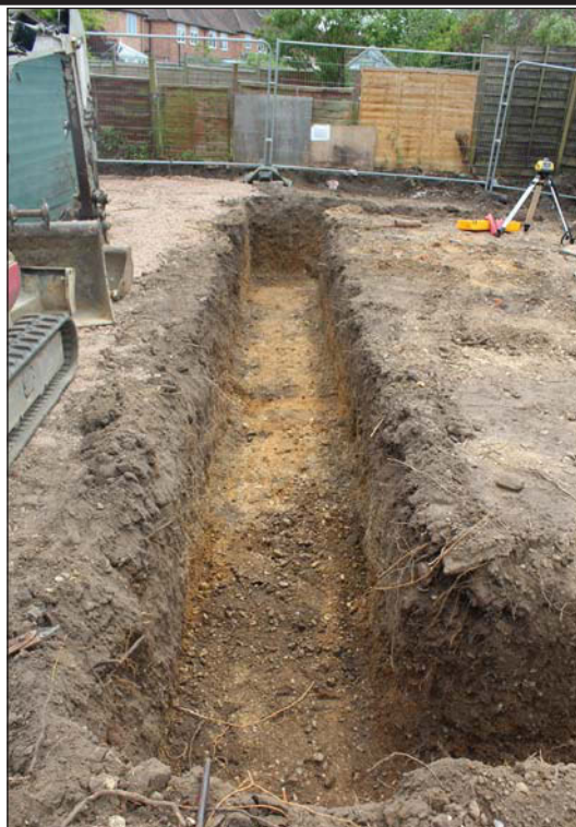
Plate 1. Eastern foundation trench, looking south-east.
