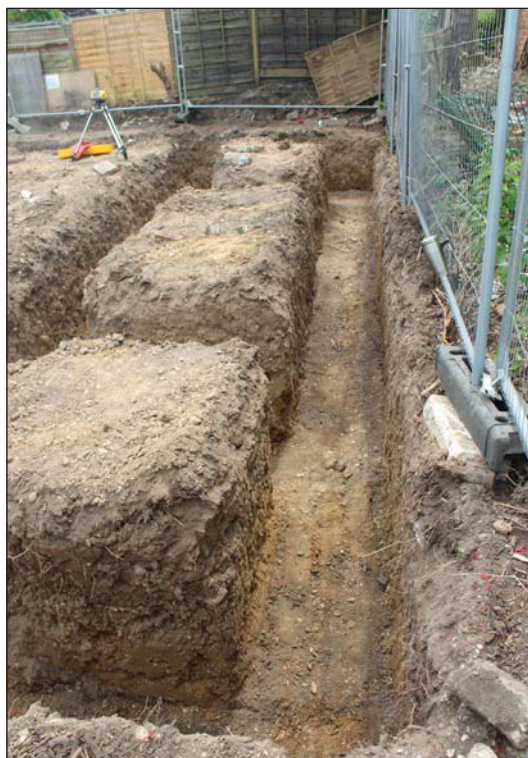
Plate 2. Western foundation trenches, looking south-east.
