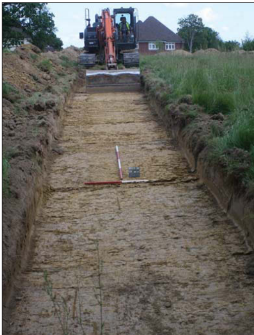
Plate 3. Trench 9, looking East. Scales: 2m, 1m and 0.50m.
