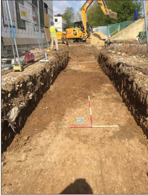
Plate 1. Northern Attenuation Tank, looking North-west. Scales: 2m, 1m and 0.50m.
