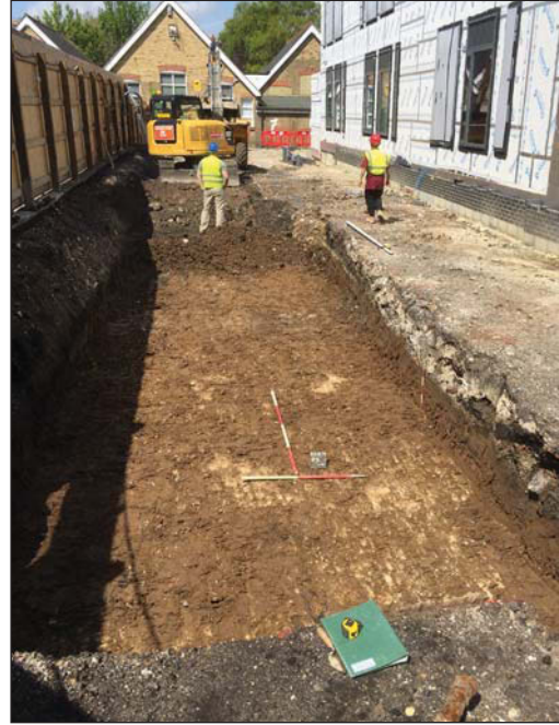
Plate 2. Southern Attenuation Tank, looking North-west. Scales: 2m, 1m and 0.50m.
