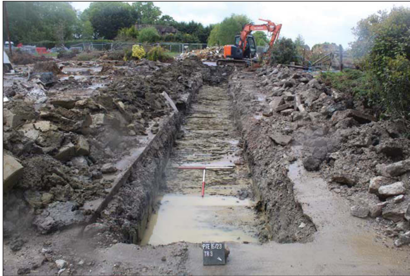
Plate 1. Trench 3, looking south west, Scales: 1m x2.
