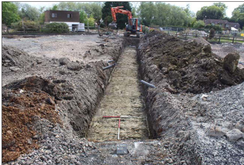
Plate 2. Trench 27, looking south west, Scales: 1m x2.
