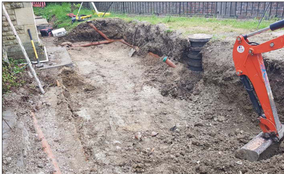
Plate 3. Excavation in progress at base of foundation level, looking north west.
