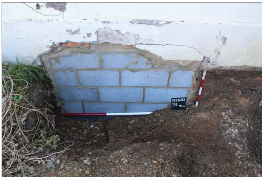
Plate 2. Blocked window in test pit 2, looking northeast, Scales: 1m and 0.5m.
