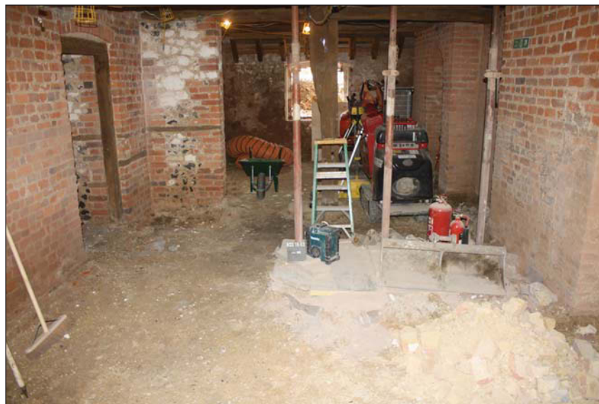
Plate 4. Interior construction, looking west.
