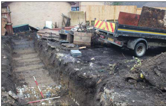
Plate 3. Trench 2, showing site conditions. Scales: 2m, 1m and 0.50m.
