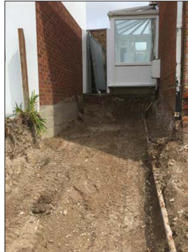
Plate 4. Area of proposed side extension, looking North.
