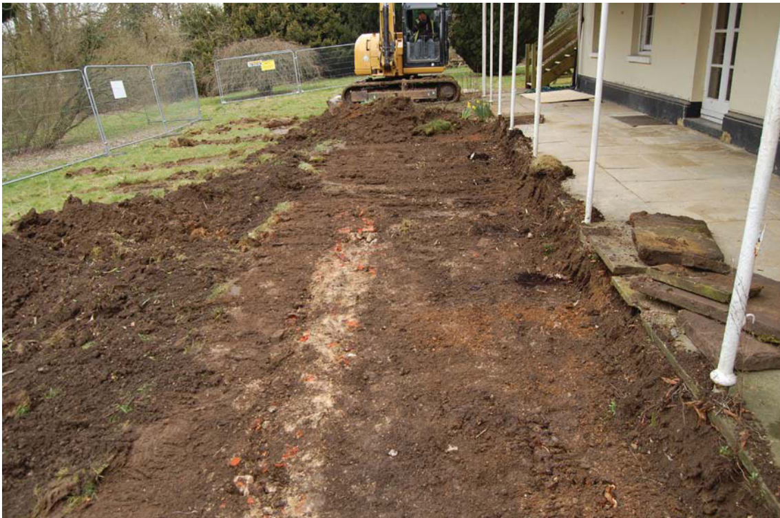
Plate 1. Strip of terrace at 0.1m deep (upper), looking north west.
