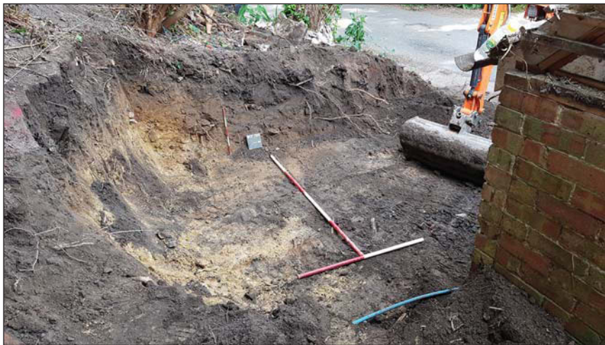
Plate 2. Site, showing bank, looking West. Scales: 2m, 1m and 0.5m.
