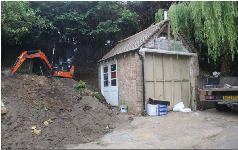
Plate 1. Site, showing existing structure, looking South-east.
