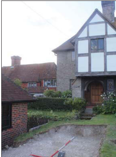
Plate 3. General view of site, looking South-east.
