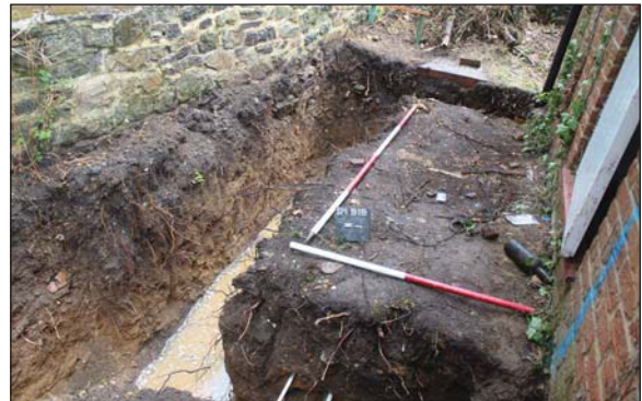
Plate 2. Footing of rear extension, looking East. Scales: 2m and 1m.
