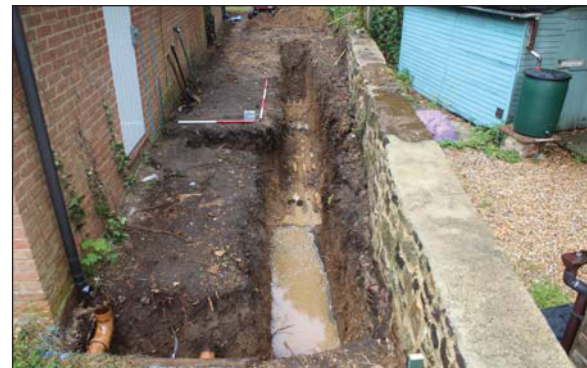
Plate 4. Footing of rear extension, looking West. Scales: 2m and 1m.
