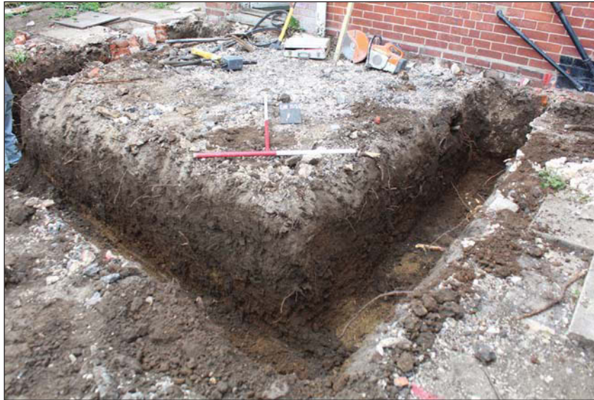
Plate 1. General view of the trench, looking north-west, Scales: 1m x2.
