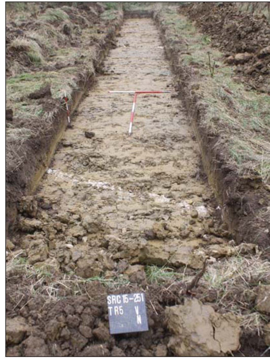
Plate 2. Trench 5, looking south, Scales: horizontal 2m and 1m, vertical 0.5m.
