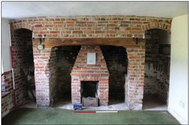
Plate 6. Room 1, fireplace, looking north-west, Scales: 2m and 1m.
