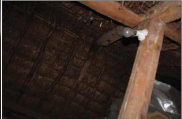
Plate 18. Roof space, truss detail.
