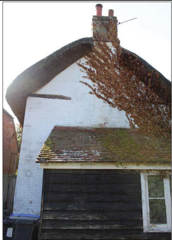
Plate 2. North-west gable end, looking south-east.
