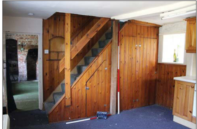
Plate 10. Room 2, looking north to stairs, Scales: 2m and 1m.
