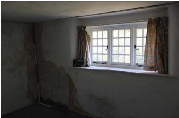
Plate 15. Room 5, looking south, Scales: 2m and 1m.
