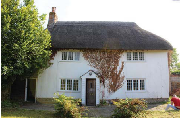
Plate 1. Front of cottage, looking north-east, Scales: 2m and 1m.
