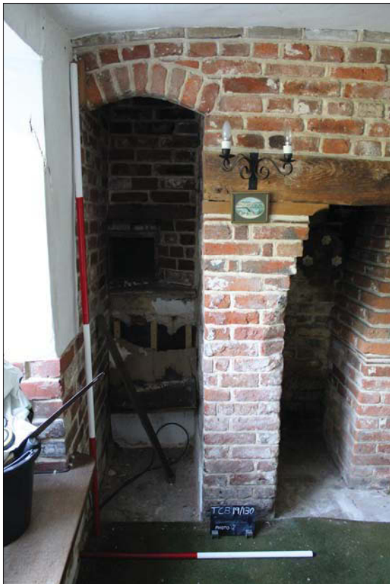
Plate 7. Room 1, fireplace alcove, looking north-west, Scales: 2m and 1m.
