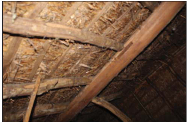
Plate 20. Roof space, purlin and common rafters.
