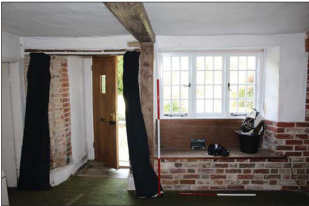
Plate 5. Room 1, looking south-west, Scales: 2m and 1m.
