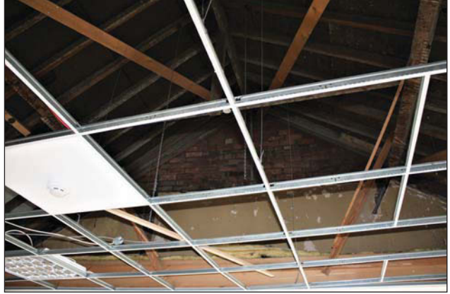
Plate 74. Second floor gable end, looking SW.
