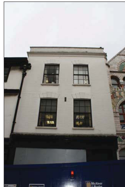
Plate 32. Exterior 36 Broad Street frontage, looking NE.
