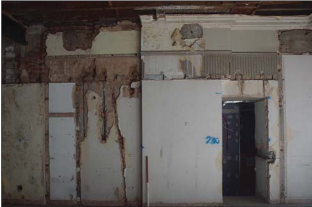
Plate 88. View to chimney breast, looking SE, Scales: 1 x 1m.
