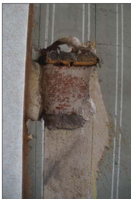
Plate 96. Fitting detail, looking NW.
