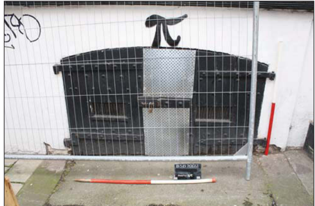
Plate 2. Exterior, undercroft entrance, 35 Broad Street, looking NE, Scales: 2 x 1m.
