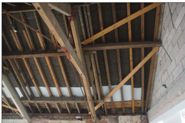
Plate 104. Roof detail showing overhanging purlin, looking NW.
