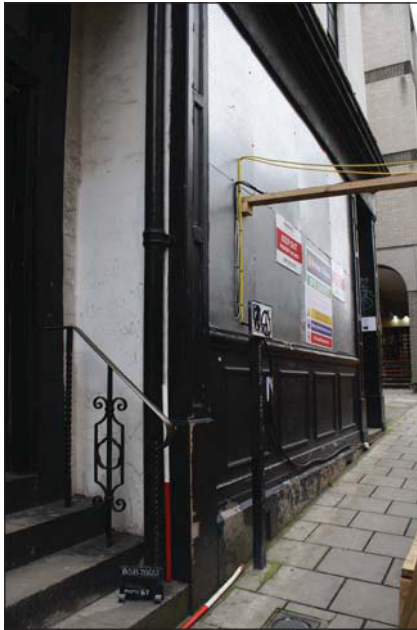
Plate 29. Exterior oblique, 36 Broad Street, looking E, Scales: 2 x 1m.
