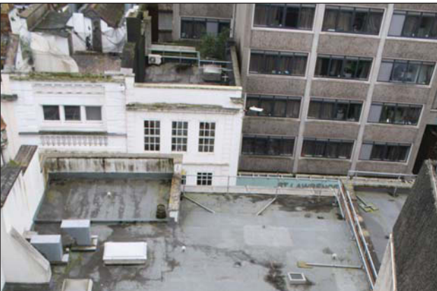
Plate 27. 35 Broad Steet roof, looking south..
