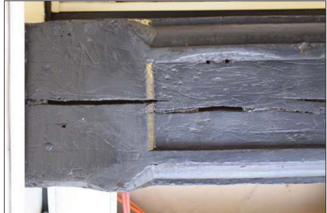
Plate 16. Ground floor beam detail, looking SE.
