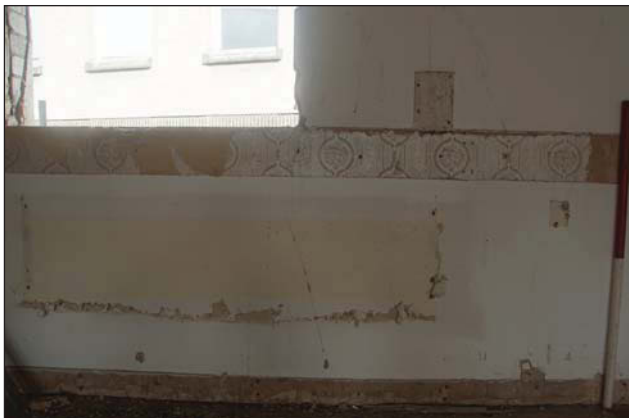
Plate 99. Wall paper detail, looking NE, Scales 1 x 1m.
