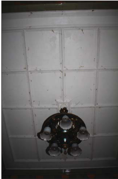
Plate 61. Ceiling detail (Everards, ground floor), looking SW.
