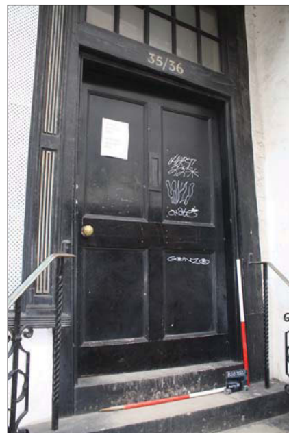
Plate 4. Exterior, door to 35 Broad Street, looking E. Scales: 2 x 1m.
