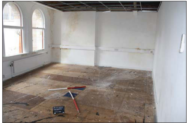
Plate 70. View to windows and blocked chimney, looking WSW, Scales: 2 x 1m.
