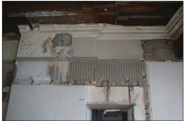
Plate 91. Picture rail and coving, looking SE.
