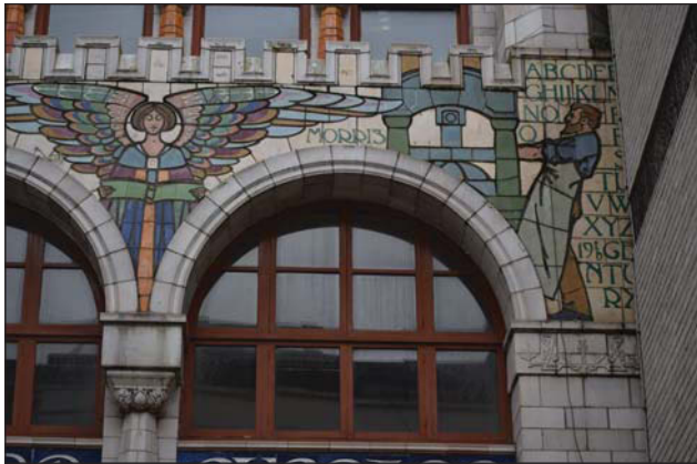
Plate 53. External, Morris detail, looking NE.
