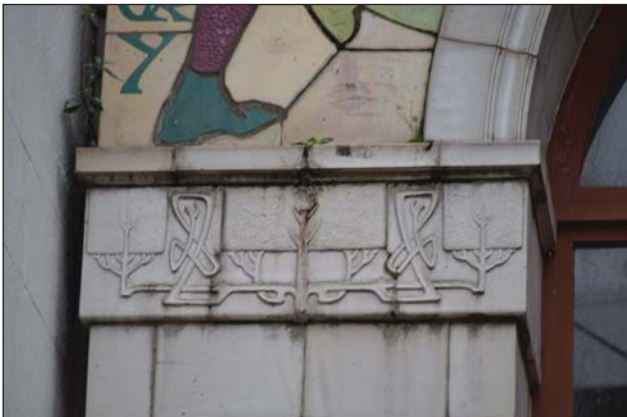
Plate 51. Exterior, Springer detail, looking NE.
