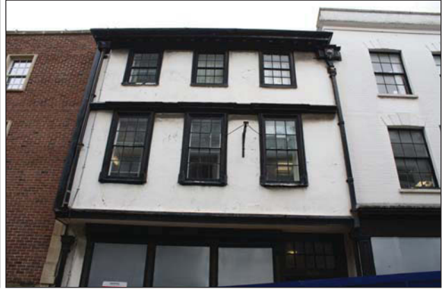
Plate 6. Exterior, frontage to 36 Broad Street, looking NE.
