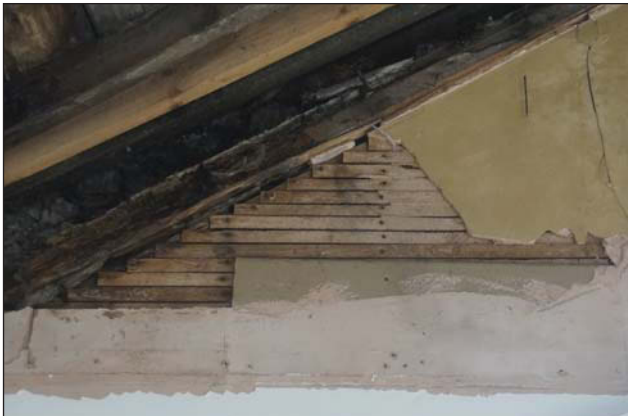
Plate 102. Gable end lath and plaster detail, looking SW.
