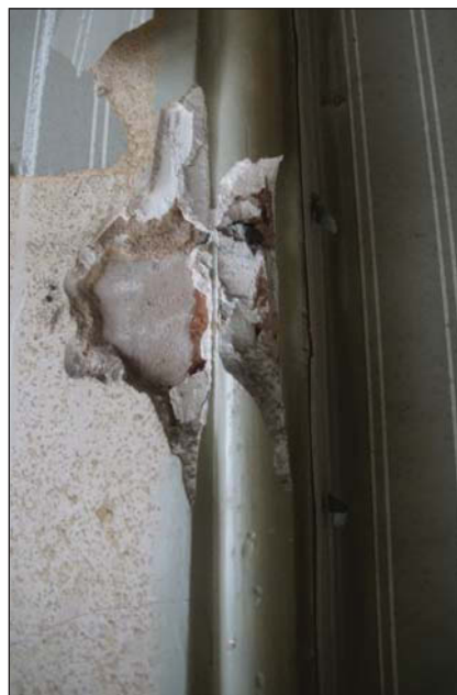
Plate 95. Chimney breast corner detail, looking W.
