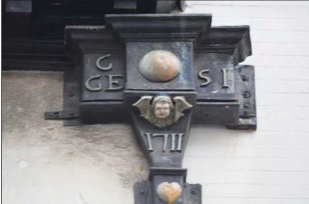
Plate 9. Exterior, hopper detail, looking NE.
