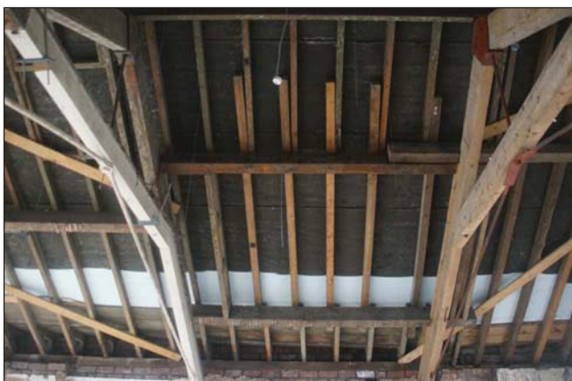
Plate 105. Roof detail, looking NW.
