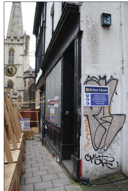
Plate 28. Exterior oblique to 36 Broad Street, looking NW, Scales: 2 x 1m.
