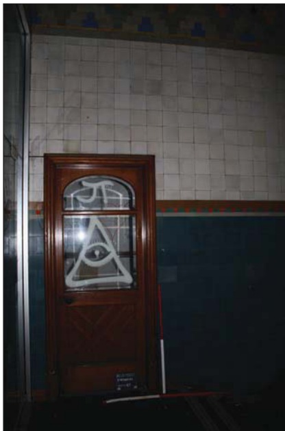
Plate 59. Ground floor door detail (Everards), looking SE, Scales: 2 x 1 m.
