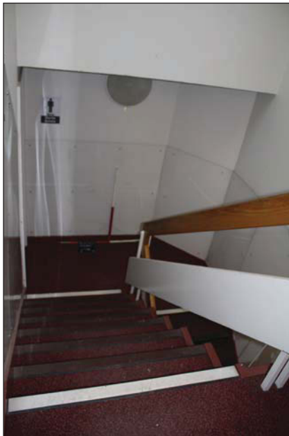
Plate 21. Second floor view stairwell, looking SE, Scales: 2 x 1m.
