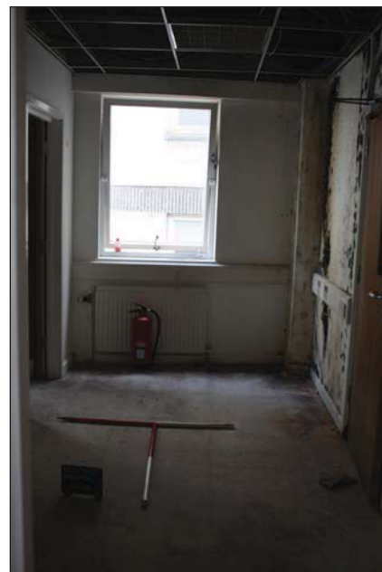
Plate 72. View along second floor corridor, looking NE, Scales: 2 x 1m.
