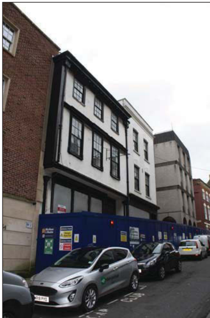
Plate 1. Exterior, oblique 35 and 36 Broad Street, looking east.
