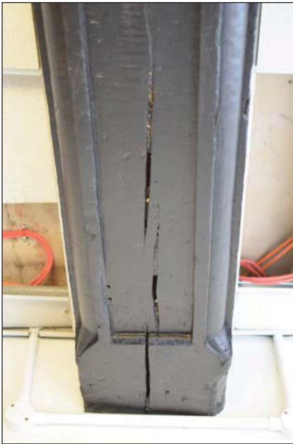
Plate 15. Ground floor beam detail, looking up.
