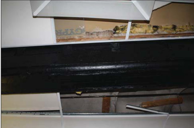
Plate 17. Ground floor, beam detail, looking NE.
