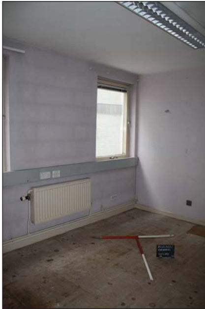
Plate 69. First floor, general view to windows , looking east, Scales: 2 x 1m.
