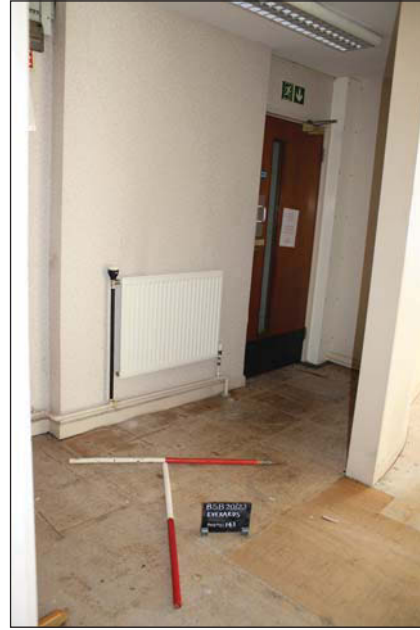
Plate 66. First floor, general view, looking SW, Scales: 2 x 1m.
