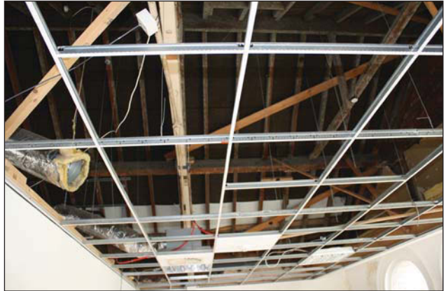
Plate 76. Second floor roof detail, looking SE.
