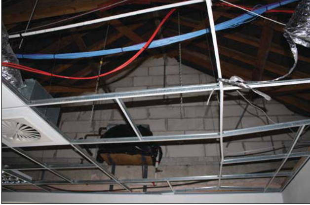
Plate 73. Second floor gable end, looking NE.
