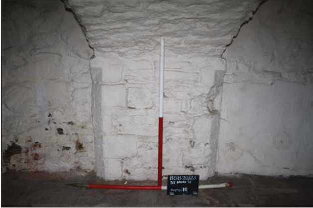
Plate 13. Lower ground 1, pier detail, looking WNW, Scales: 2 x 1m.
