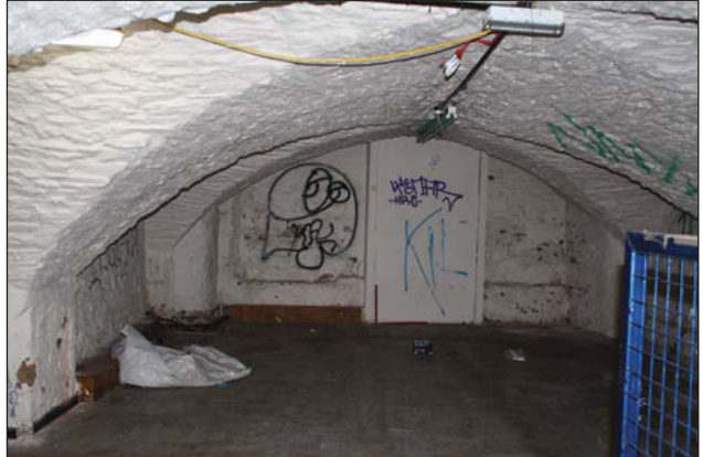
Plate 10. View to blocked door, lower ground 1, looking SW, Scales: 2 x 1m.
