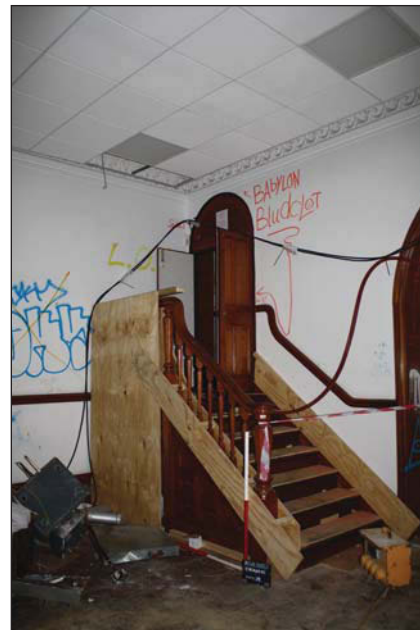
Plate 64. Stair detail (Everards, ground floor), looking SW, Scales: 2 x 1m..
