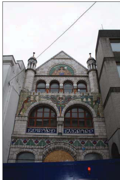
Plate 48. Exterior, frontage to Everards, looking NE.
