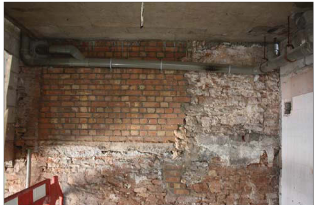
Plate 85. Lower half of arch, looking SE.
