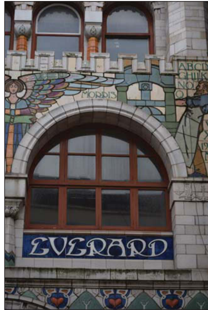
Plate 50. Exterior, Everard window detail, looking NE.
