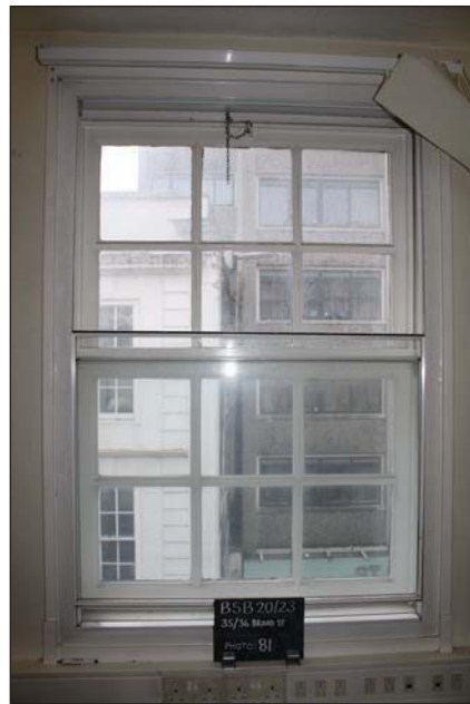
Plate 8. Second floor window detail, looking SW, Scales: 2 x 1m.
