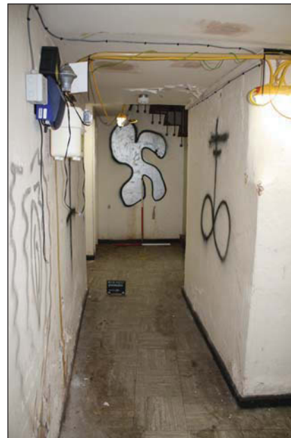
Plate 36. View along corridor, lower ground 1, looking W, Scales: 2 x 1m.
