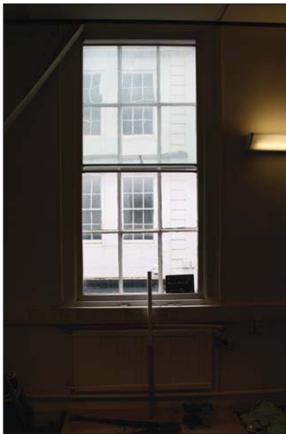
Plate 7. First floor window detail, looking SW, Scales: 2 x 1m.
