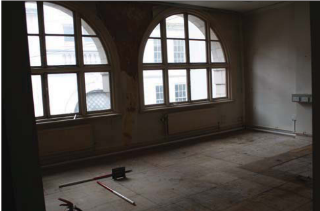
Plate 67. First floor, view to windows, looking W, Scales: 2 x 1m.
