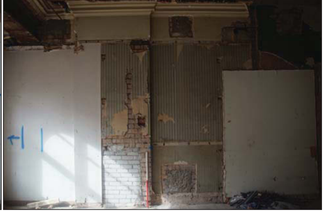
Plate 87. View to chimney breast, looking NW, Scales: 1 x 1m.
