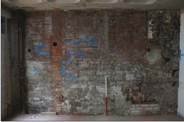
Plate 86. Wall detail showing brick area, looking SE, Scales 1 x 1m.
