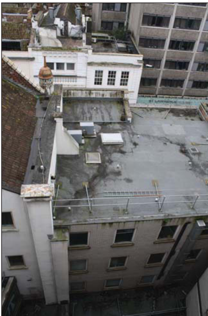
Plate 43. 36 Broad Street roof, looking south.
