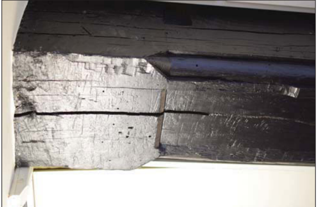
Plate 18. Ground floor, beam detail, looking NE.
