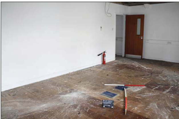
Plate 71. Second floor, general view, looking east, Scales: 2 x 1m..
