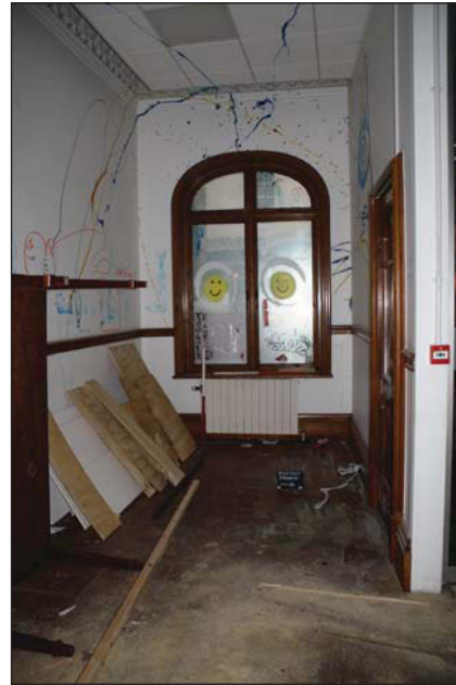
Plate 62. View to window (Everards, ground floor), looking SSE, Scales: 2 x 1m.
