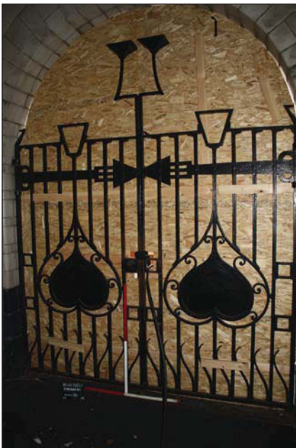
Plate 47. Ground floor, Everards gate detail, looking SW, Scales: 2 x 1m.
