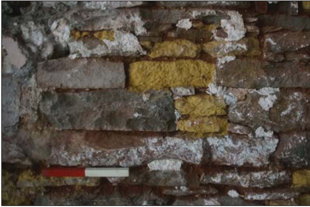
Plate 82. Wall detail, looking SE, Scales 1 x 0.2m.
