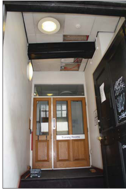
Plate 14. Ground floor, entrance lobby, looking NW, Scales: 2 x 1m.
