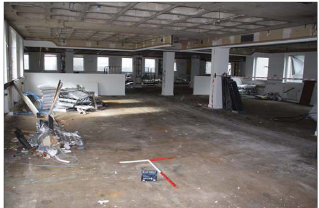
Plate 80. Second floor general view, looking North, Scales: 2 x 1m.
