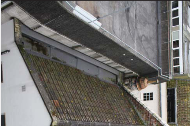
Plate 75. Everards roof, looking SW.
