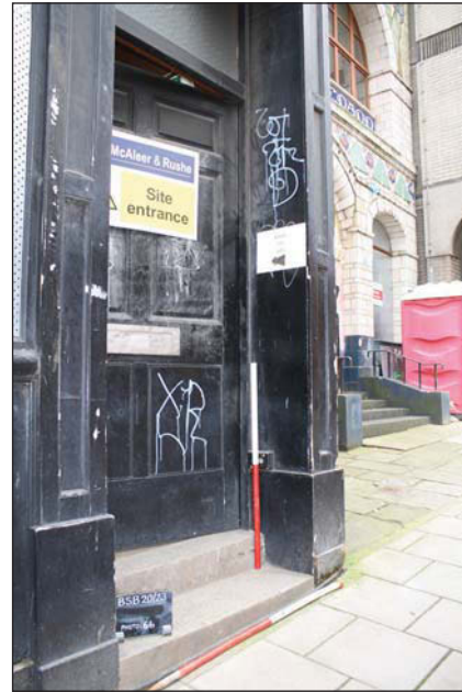
Plate 30. Exterior Door, 36 Broad Street, looking NE, Scales: 2 x 1m.
