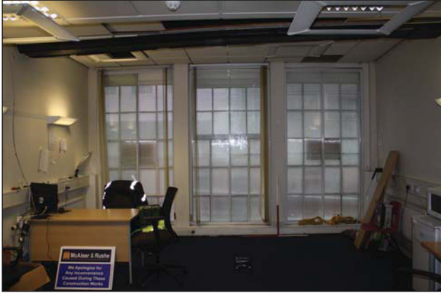
Plate 5. Ground floor, view to windows, looking SW, Scales: 2 x 1m.
