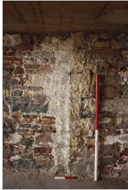
Plate 83. Stone quoins, looking SE, Scales: 0.2m & 1m.
