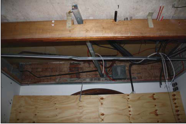
Plate 65. Brickwork above arch (ground floor, Everards), looking east.
