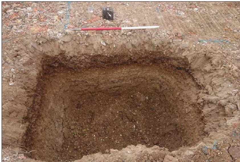
Plate 2. Pile cap 80, looking south east, Scales: 1m.
