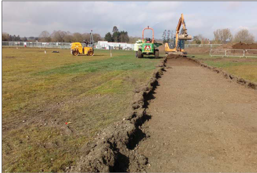
Plate 1. Access strip (topsoil only), looking north east.
