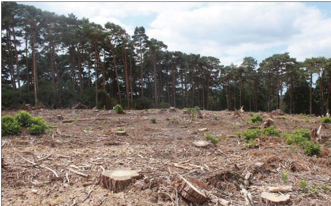
Plate 2. Phase 2 during earthwork walk over after rhododendron removal and tree felling
