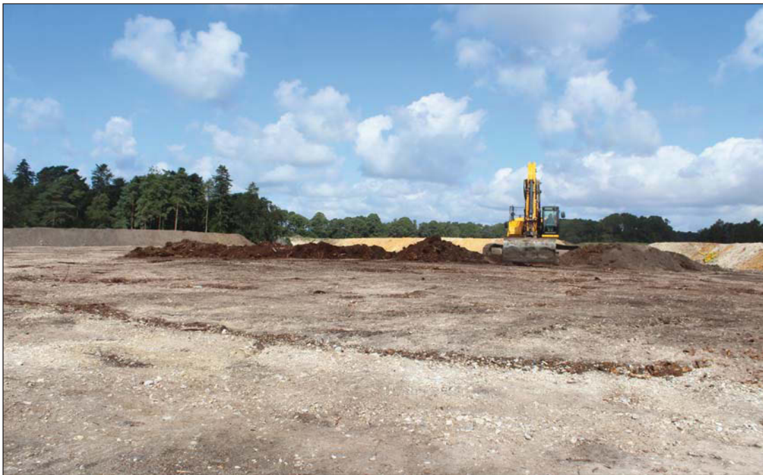
Plate 4. Phase 2 looking west whilst topsoil stripping
