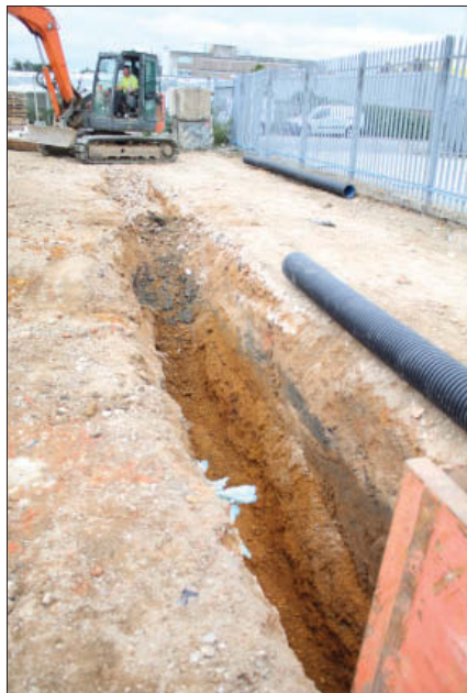
Plate 3. Pipe trench, western boundary, looking SW.
