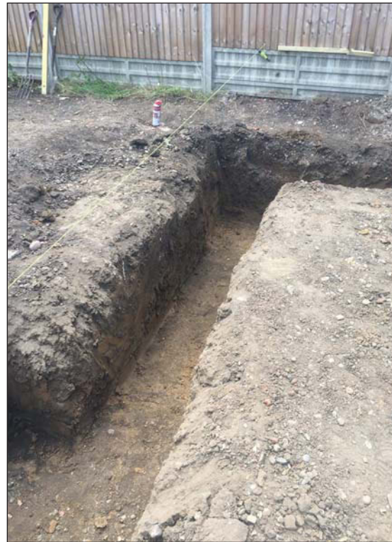
Plate 2. South footing in south west corner, looking west.
