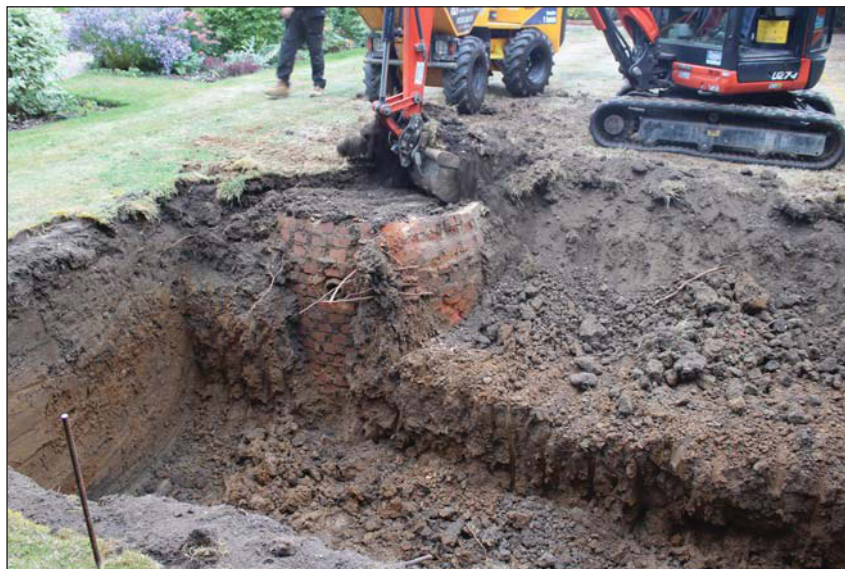
Plate 4. The Victorian well or soakaway, looking NW
