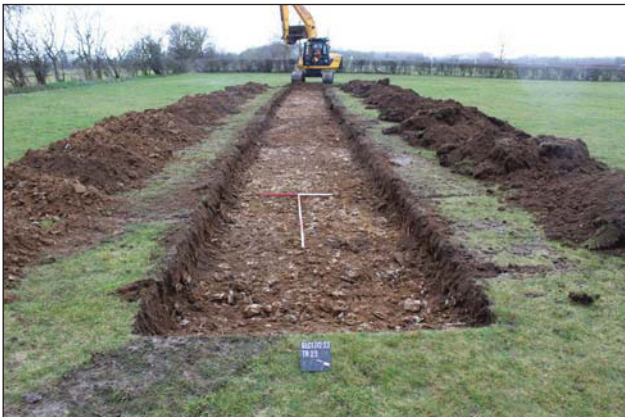
Plate 7. Trench 23, looking WSW, Scales: 2m and 1m.
