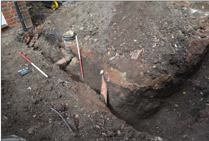
Plate 1. Excavation south footing, with modern services, looking north-west, Scales: 1m x2.
