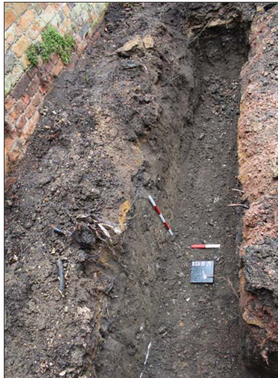
Plate 2. Eastern footing at base of 19th century wall, looking south, Scales: 0.5m and 0.1m.
