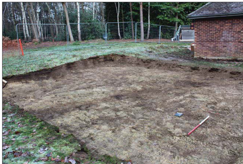
Plate 2. Initial stripped area south of existing building looking West. Scale: 1m.
