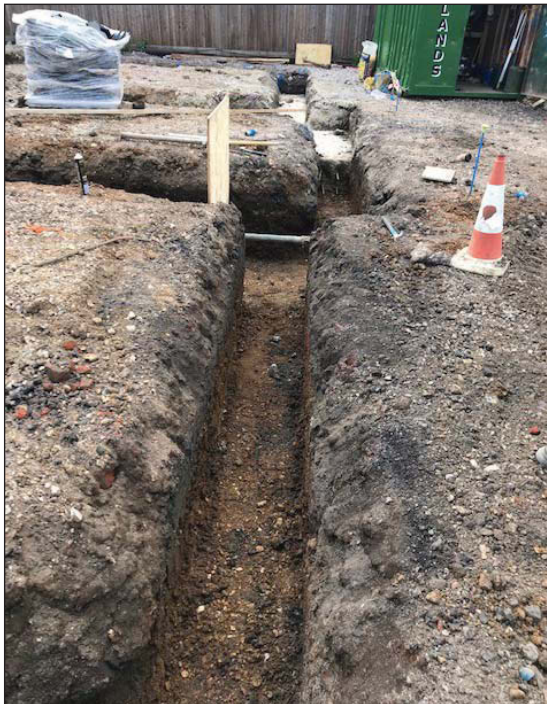
Plate 4. Plot 3 foundation trench looking south (from client).
