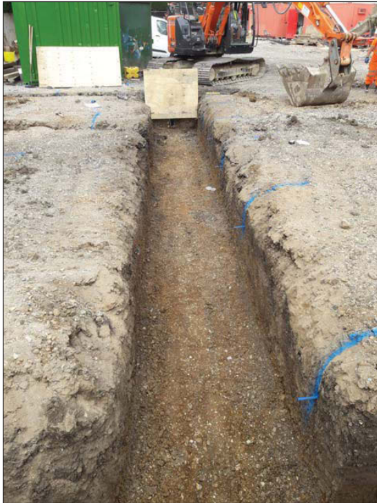
Plate 3. Plot 3 foundation trench looking west (from client).
